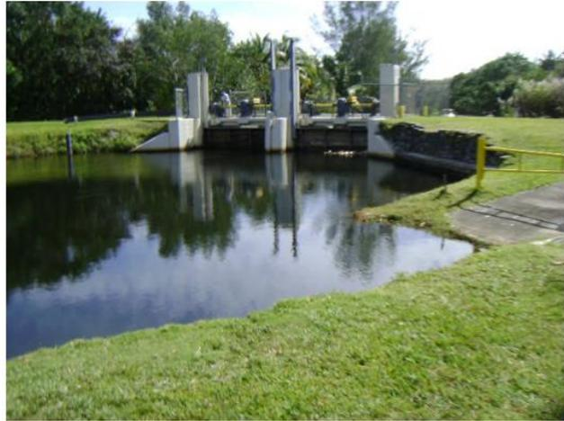
The project consists of enhancing the S-22 Coastal Structure and installing forward pumps to increase its resiliency and maintain basin discharge levels while sea levels rise. The SFWMD has developed advanced H&H models to evaluate system operations under changed current and future conditions and recommended infrastructure investments in critical locations. Recent observations and model results show that the S-22 Structure needs adaptation.
