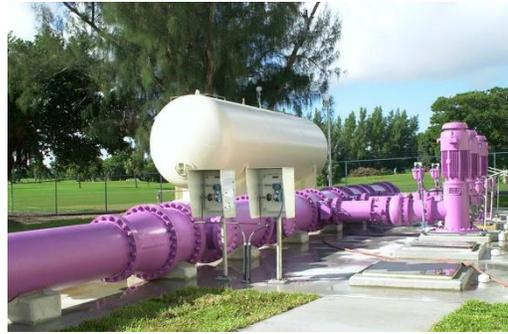
Figure 9. Picture of reclaimed water "purple pipes".
