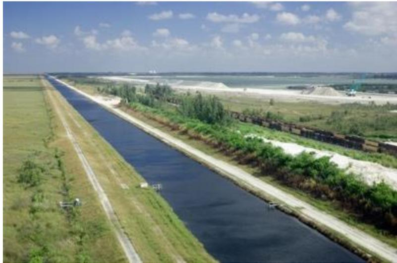
Funds are needed to advance resiliency strategies to reduce vulnerability of communities upstream of the L-31E Levee. Future modeling efforts will determine additional resiliency needs at other levee structures, based on the determination of what cross sectional change that a vulnerable levee would need to provide more protection from storm surge and SLR.
