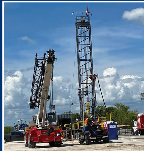
Test/Exploratory Well Drilling at C38S
