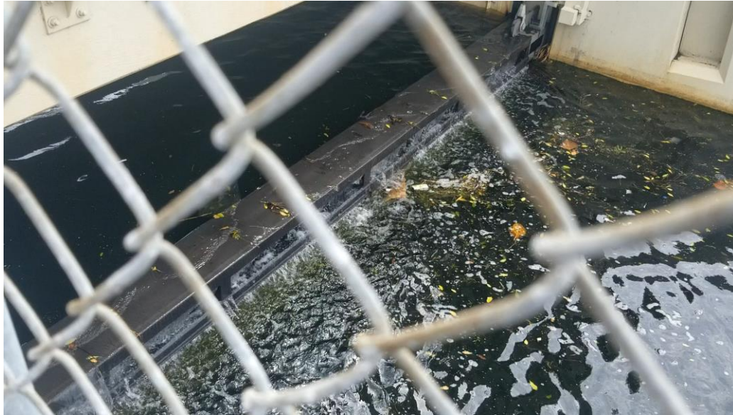
October 2019: Gates closed, high tide water reverse flowing over the top of the gate
