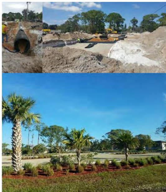
Figure 4-9: Felts Avenue Bioreactor Bonita Springs 14
