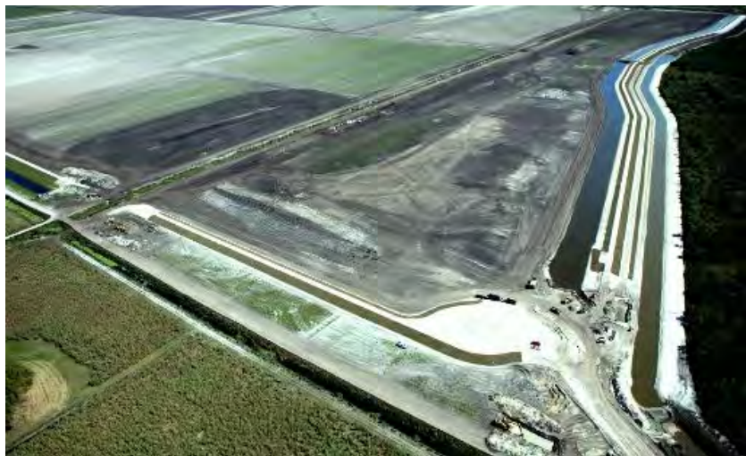
Figure 4-3: Spreader Berms and Canals
