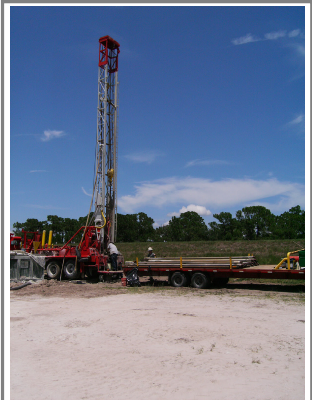
Applied Drilling Engineering drilling the 17-inch pilot hole
