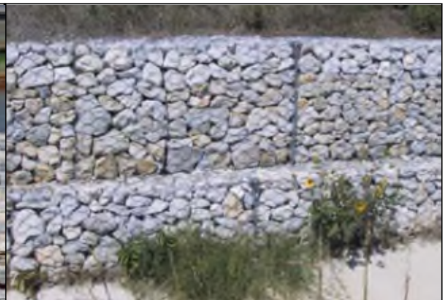
Figure H2. Bank stabilization with gabion baskets (from NRCS 3 , 2007)
