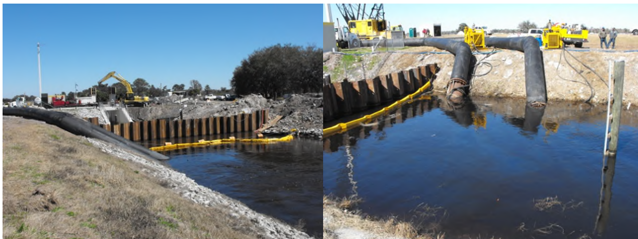
Figure G2. Temporary pump station at S-60 (head water at right, tail water at left)
