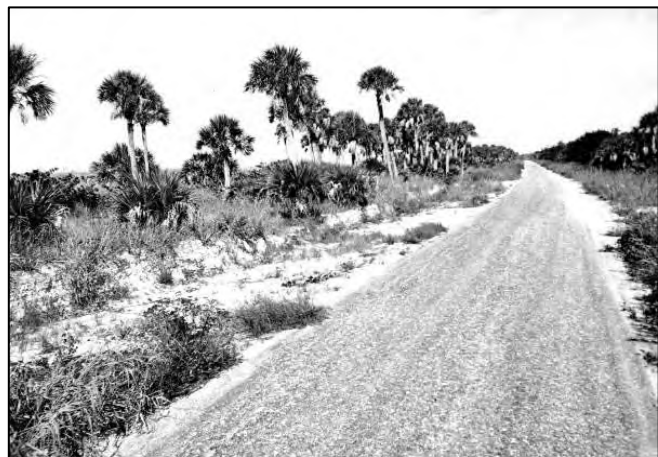
Figure 5. Road from Naples to Gordon Pass circa 1935 (State Library & Archives of Florida).
