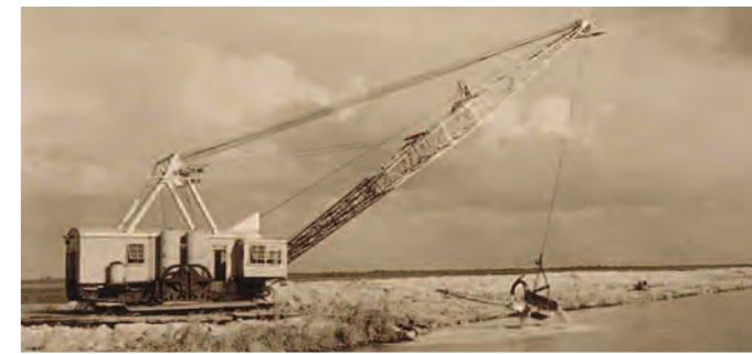
A world class flood control project was started in the early 1950s to effectively drain floodwaters from Florida and protect its residents. This dragline is shown in 1955. Construction of the project continued into the 1970s.
