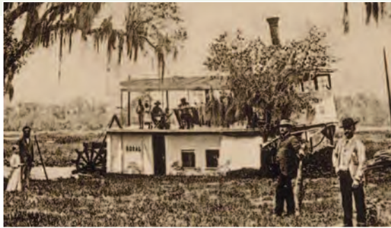
The first canal draining water from Lake Okeechobee was built in the 1880s. These canals later allowed successful steamboat travel on the lake and associated rivers.
