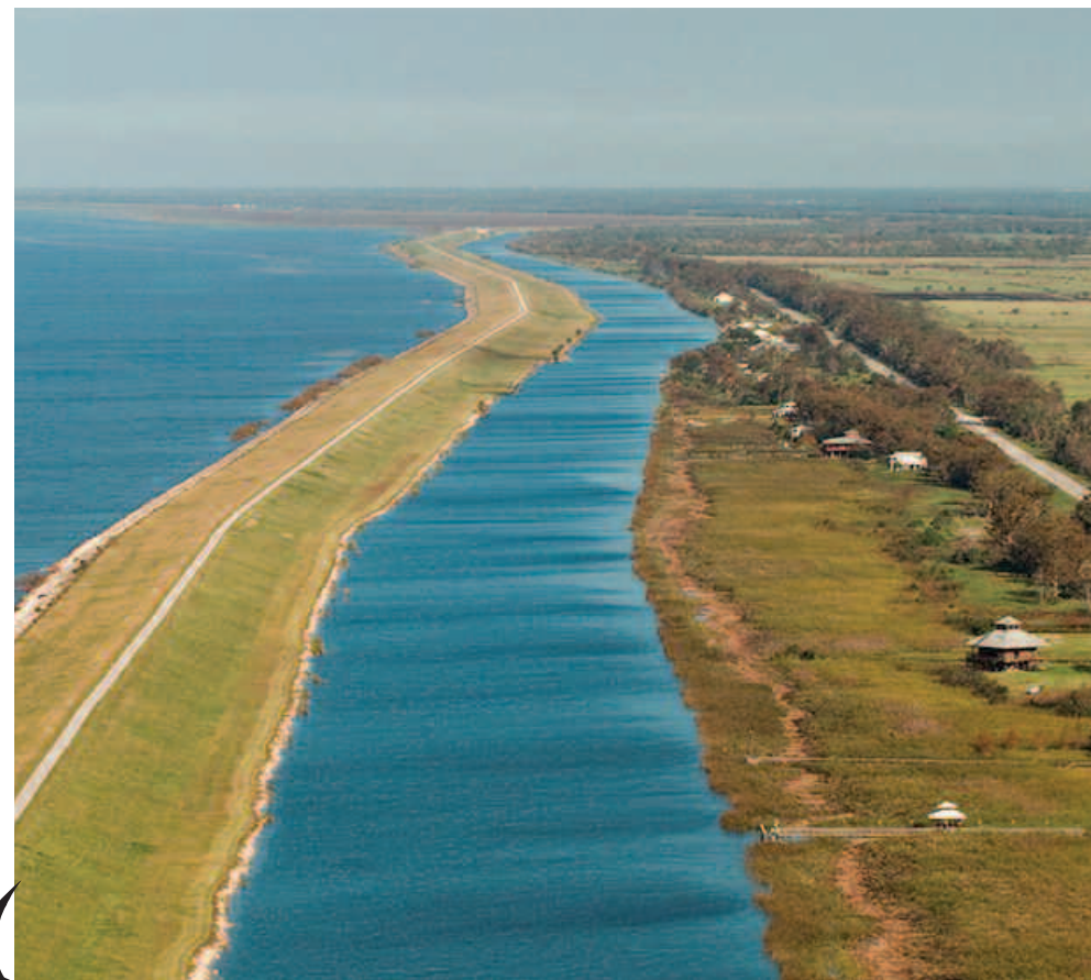
From left: Lake Okeechobee, the Herbert Hoover Dike, the rim canal, and the shoreline.
