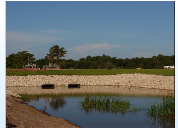
S-67 water control structure (replaced G-85 structure) Source: SFWMD
