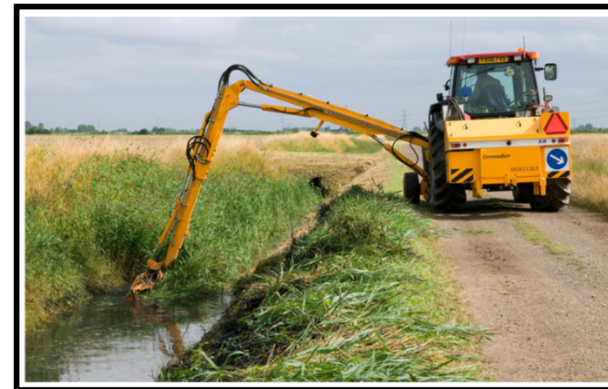
Mechanical Ditch Cleaning
