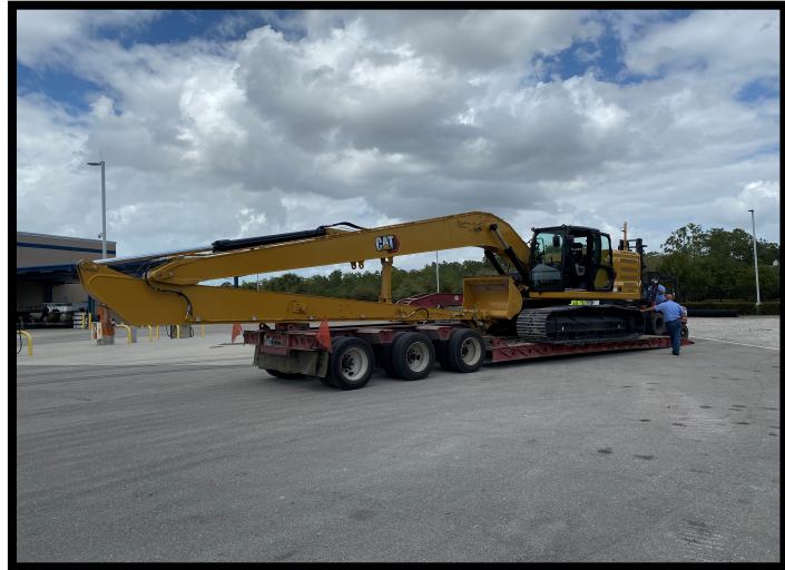
Long Reach Excavator
