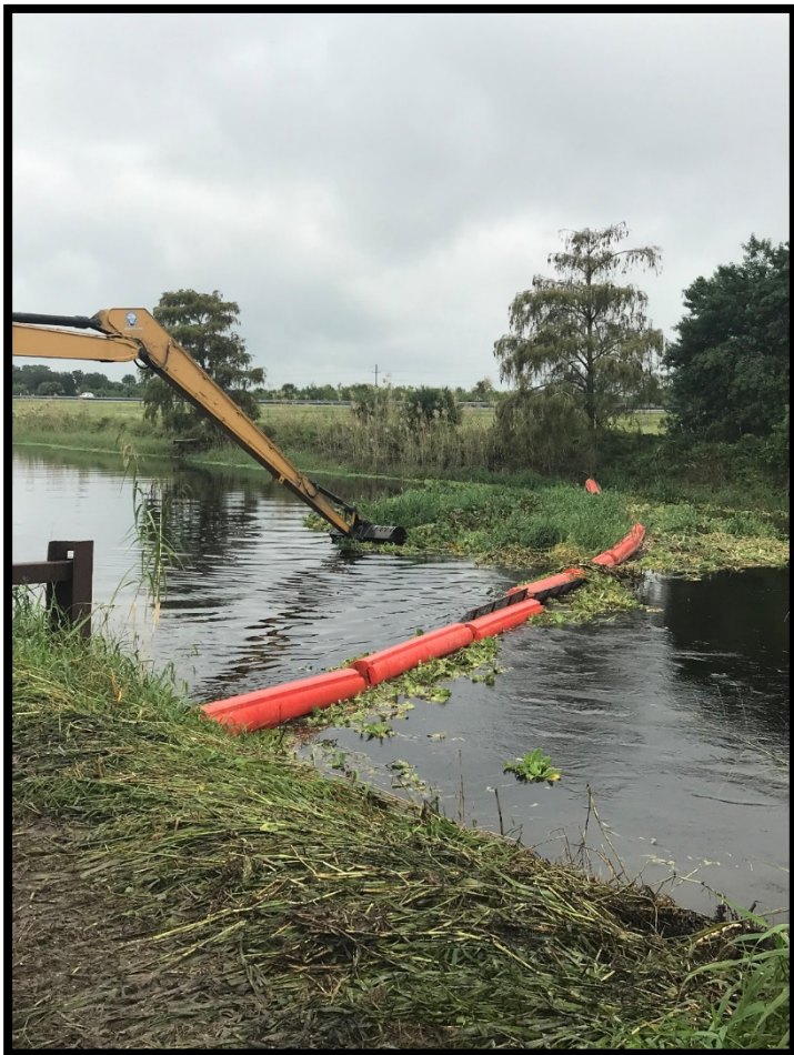
Mechanical Removal of Vegetation From Barrier
