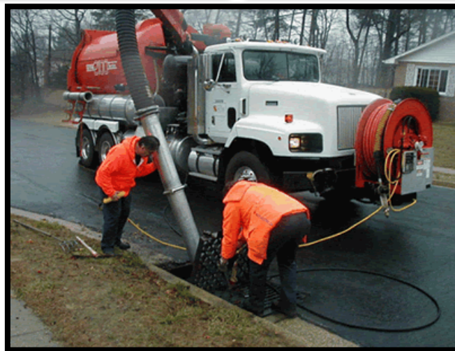
Storm Drain Cleaning
