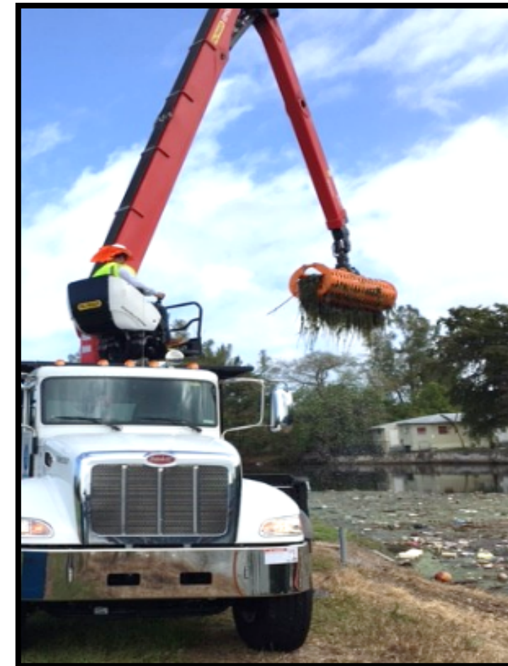
Mechanical Removal of Debris From Barrier
