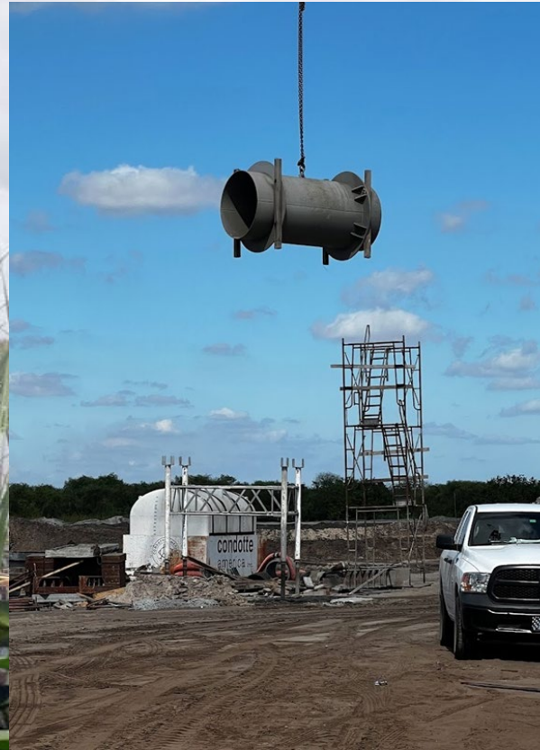
Pump Housing Placement
