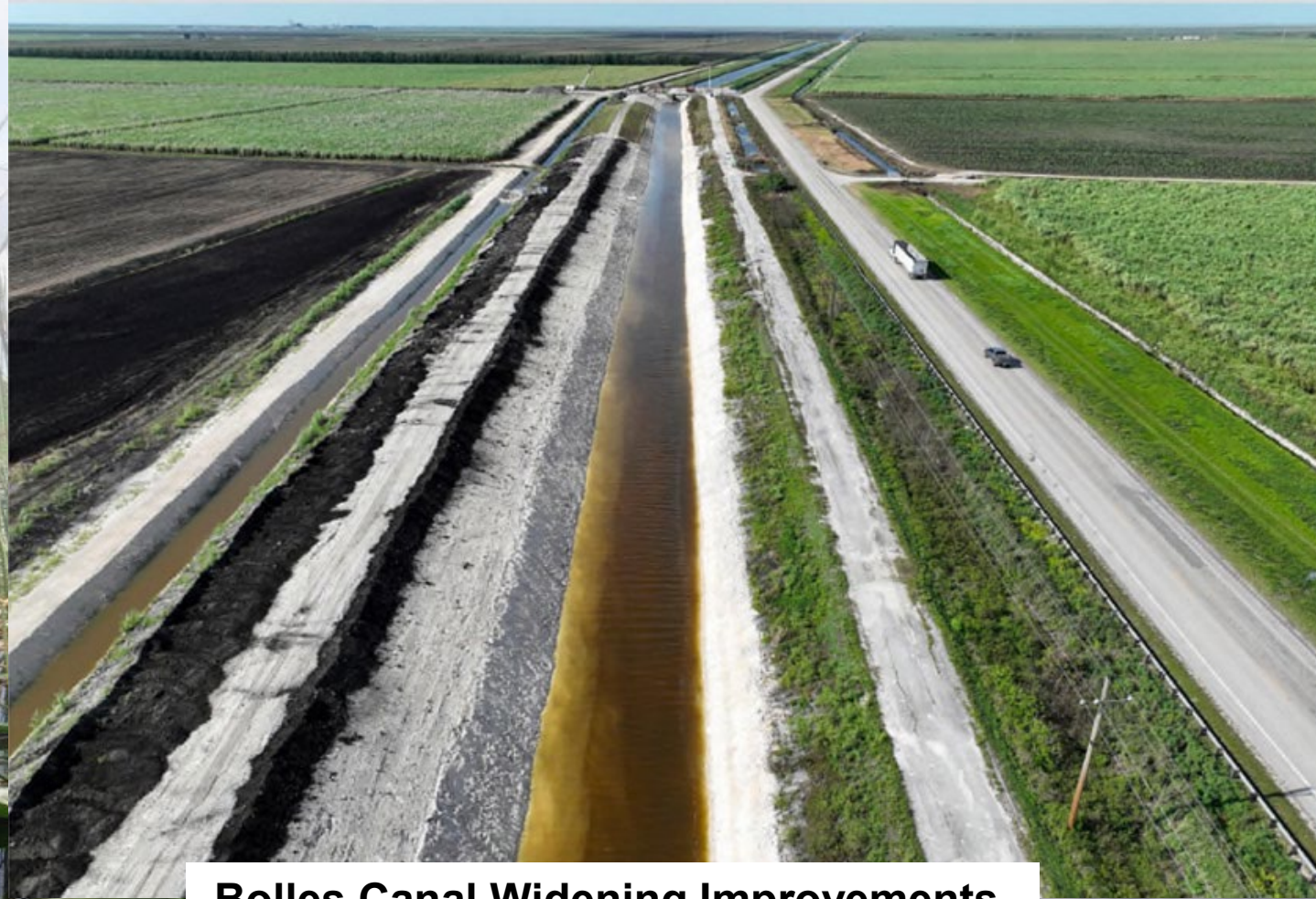
Bolles Canal Widening Improvements
