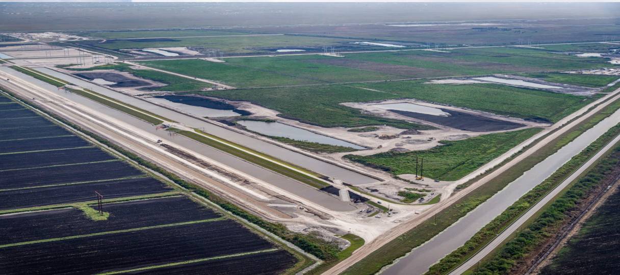
North Inflow Canal and Levee
