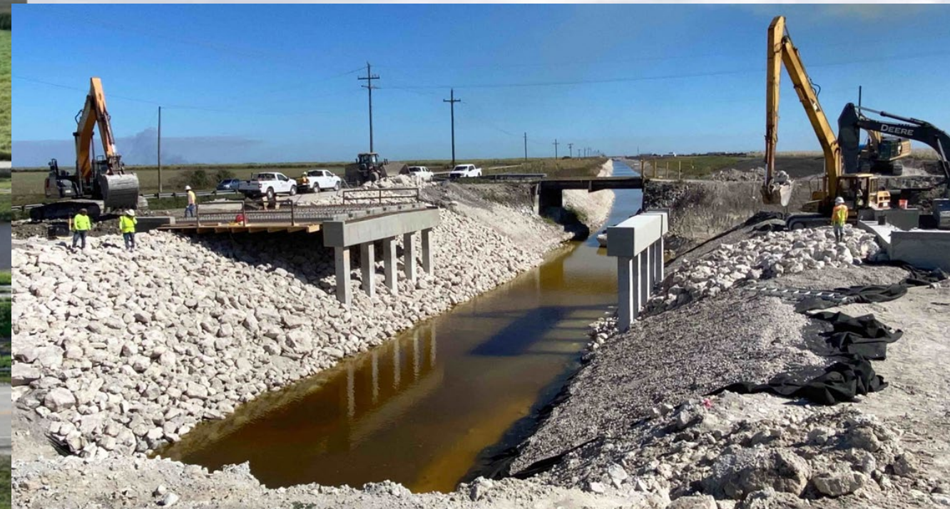
FDOT Beam Slab Placement
