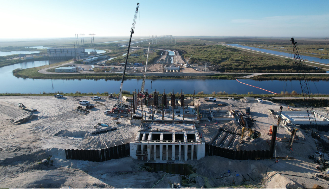
G-780, Dissipator & Lined Discharge Channel
