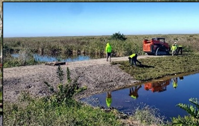
STA-2 Cell 2 East Borrow Canal Restoration of 37 Canal Plugs – 15 Complete
