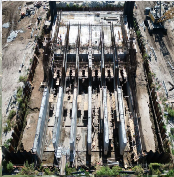
G-550 Pump Station Concrete & Reinforcement
