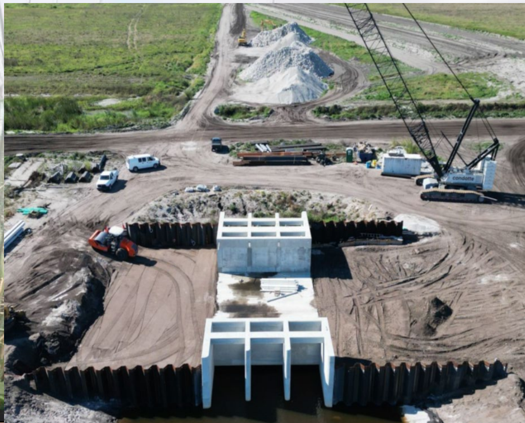
G-551 Outflow Structure 100% Concrete Completed
