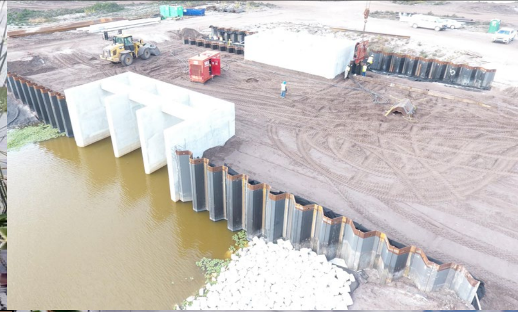
Eastern Levee construction over the G-551 Outflow Structure nearing completion
