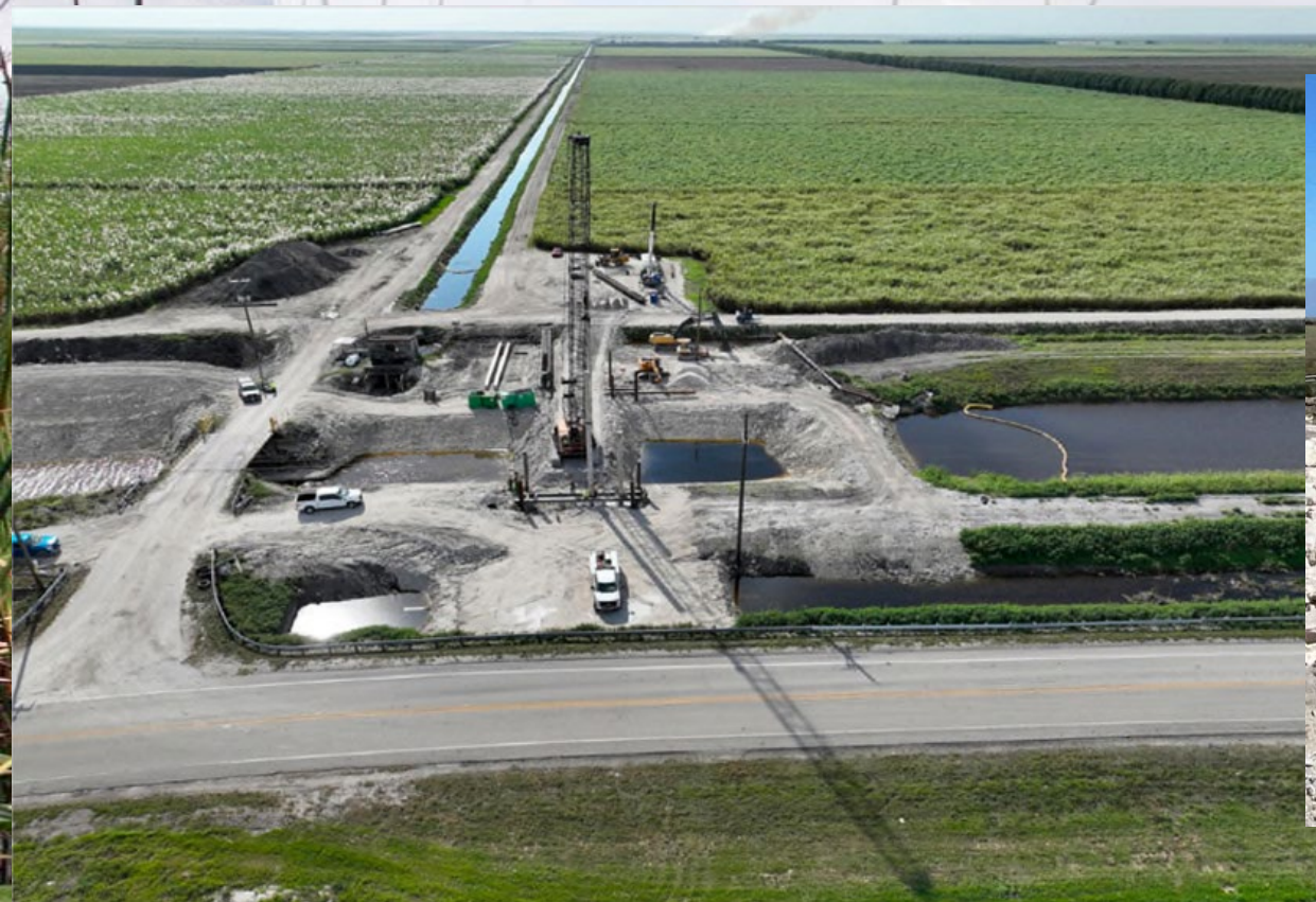
Pile Placement Star Farm Bridge
