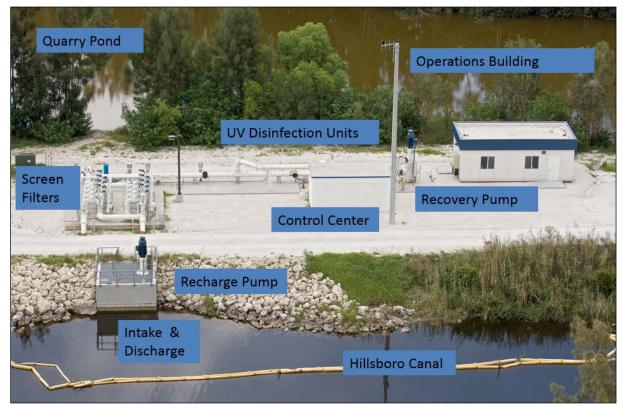
Figure 2. Aerial view of the constructed Hillsboro ASR system.
