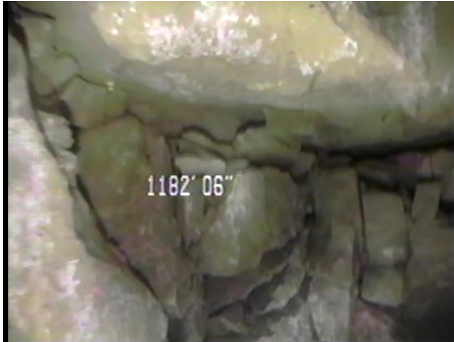
Figure 4-6. BHV view of large cavity in OSF-105 (1,182 ft bls).
