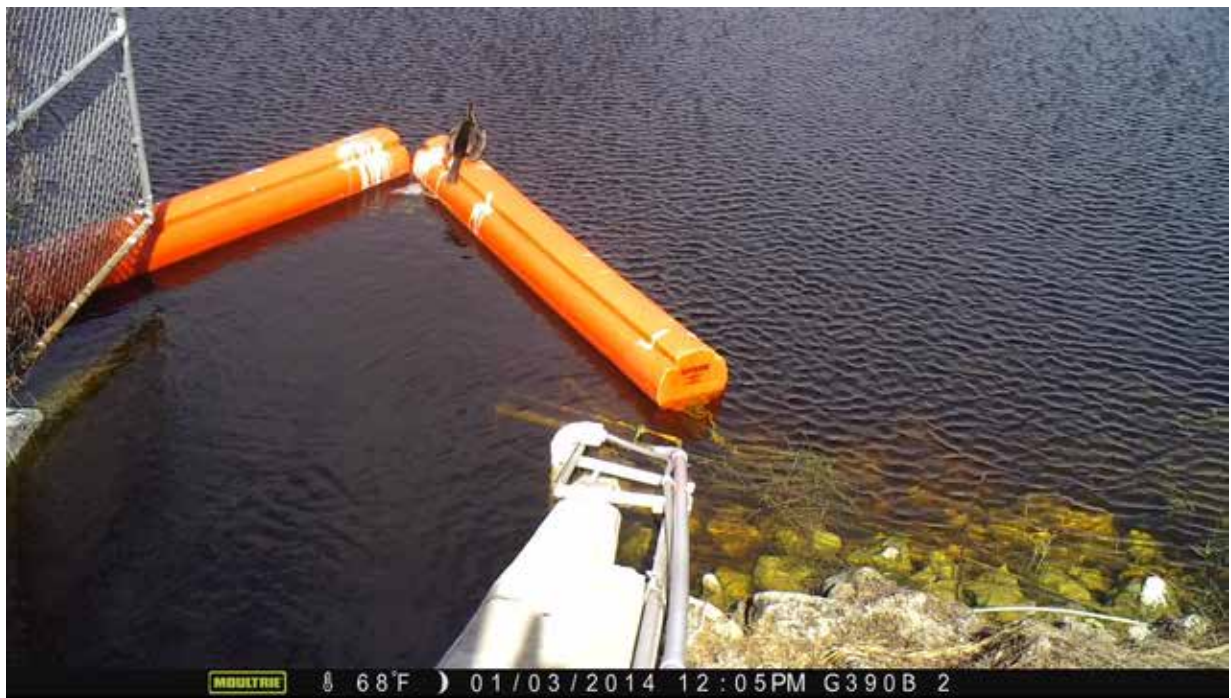
Figure 5. Sampling equipment at G390B mounted on the structure wing wall.
