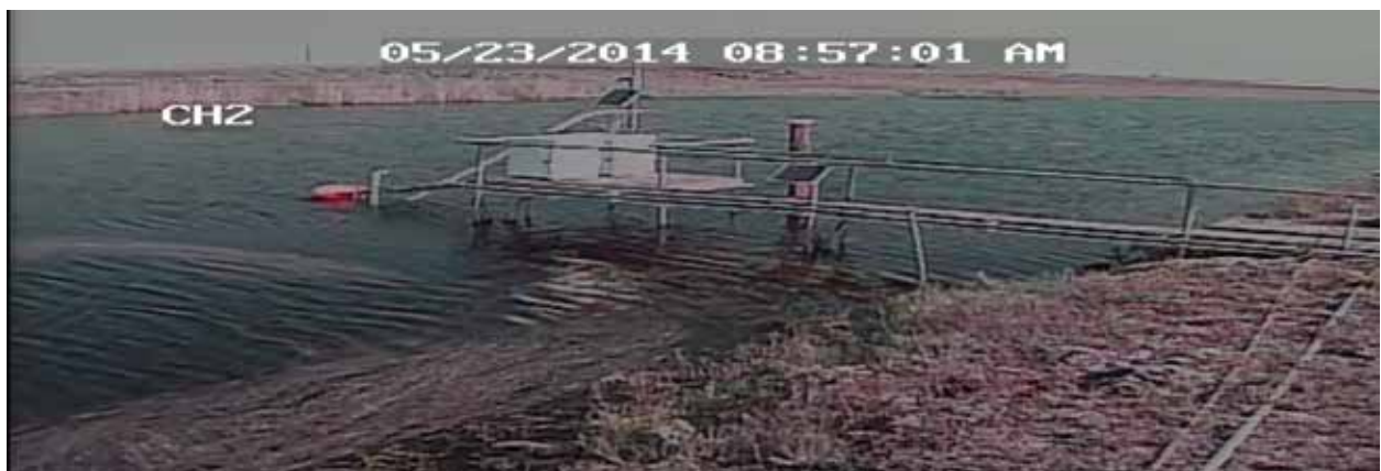
Figure 10. G310 on the morning of May 23, 2014, showing the arrival of uprooted cattail from downstream of the platform.
