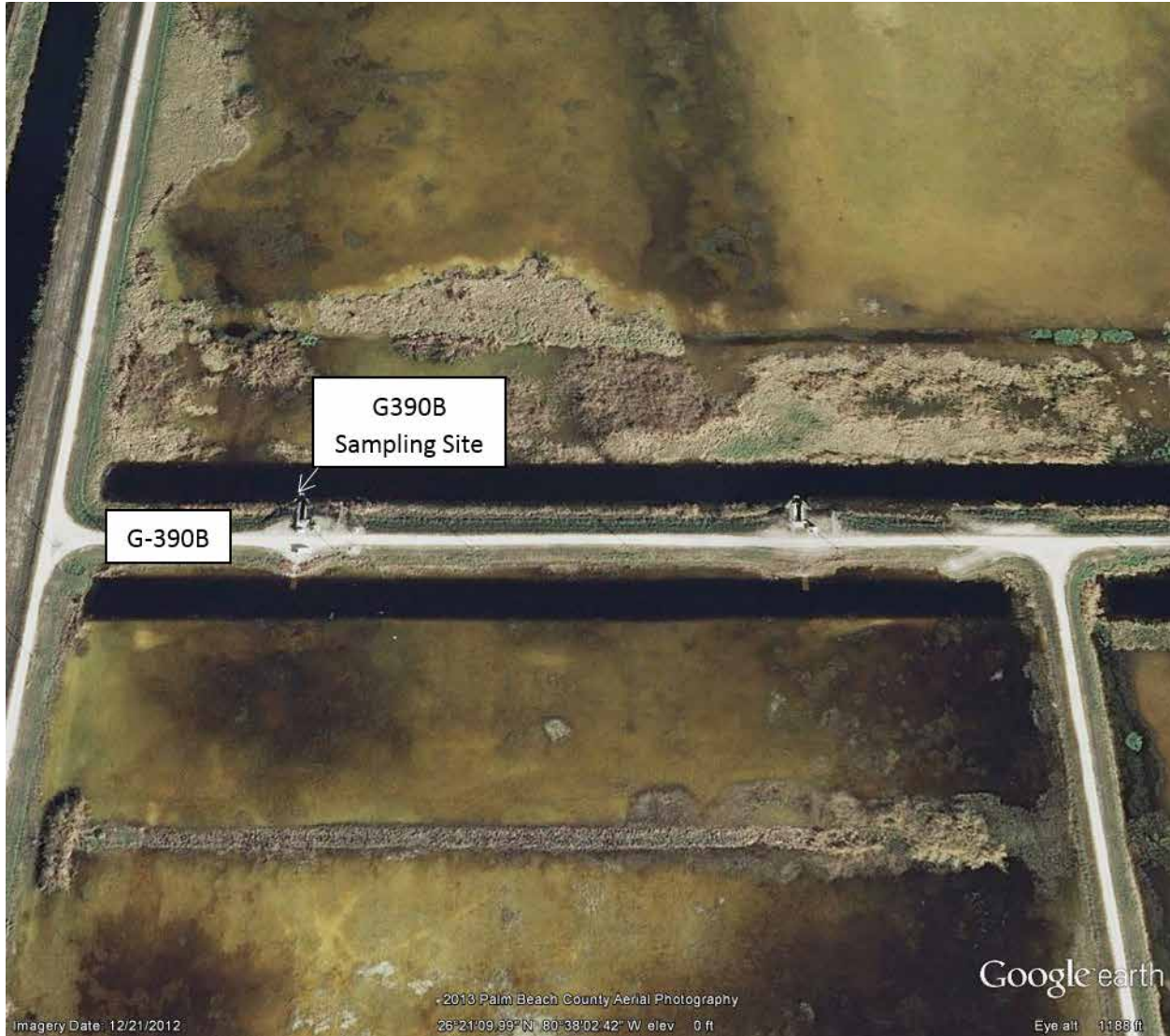
Figure 2. Structure G-390B, the inflow to the Periphyton-based Stormwater Treatment Area Project, and the G390B sampling site.
