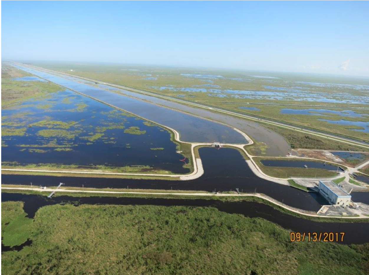
Figure 10. East Seepage Zone Canal on September 13, 2017.
