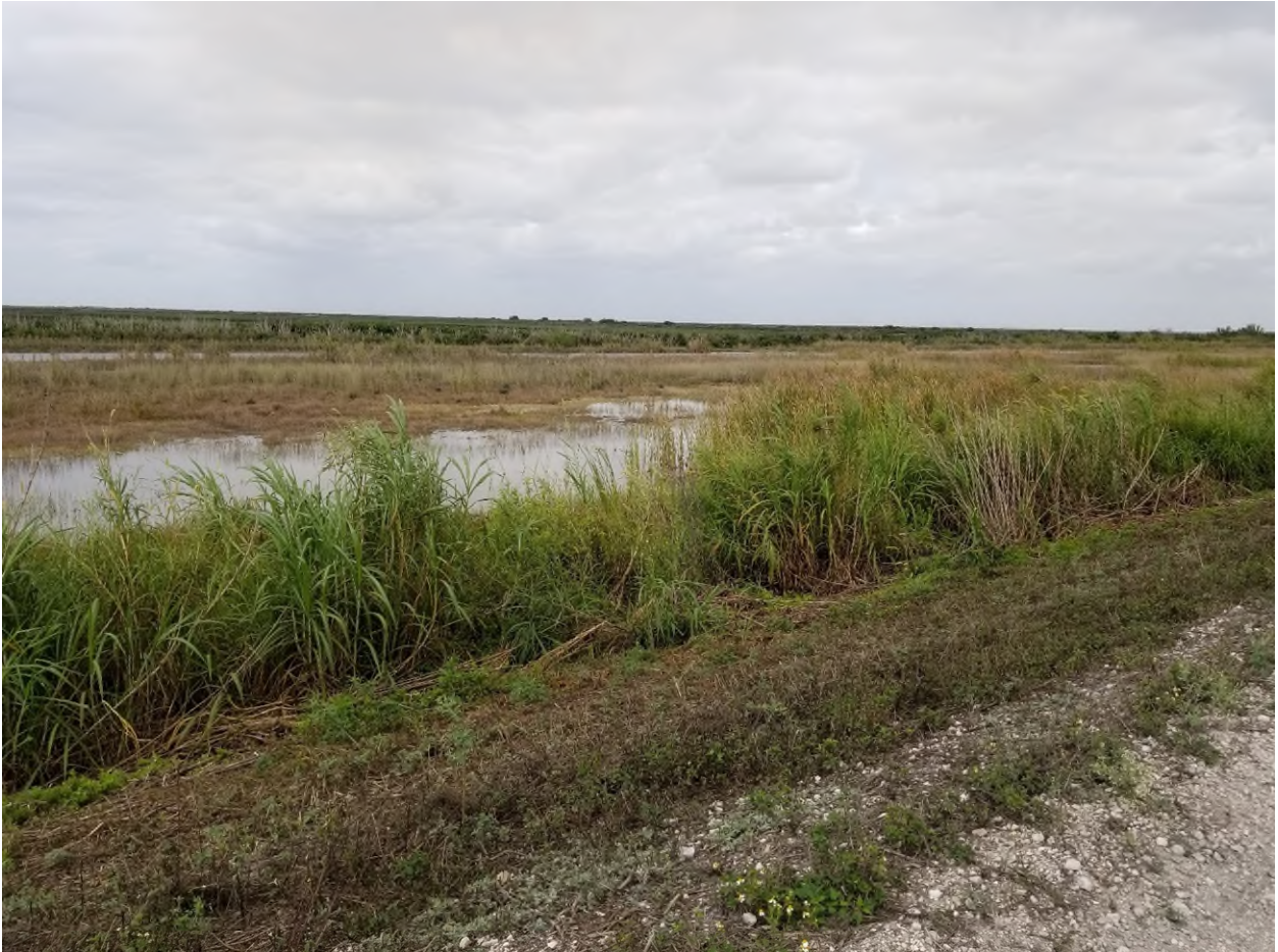
Figure 9. Wet area outside North/Northwest Seepage Zone on February 22, 2018.
