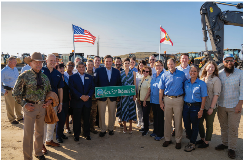
Governor Ron DeSantis, along with state and local officials, breaks ground on embankments and canals to advance the Caloosahatchee (C-43) Reservoir.
