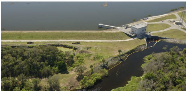
Figure 12. Ten Mile Creek, WPA, and pump station. (Photo by SFWMD.)
