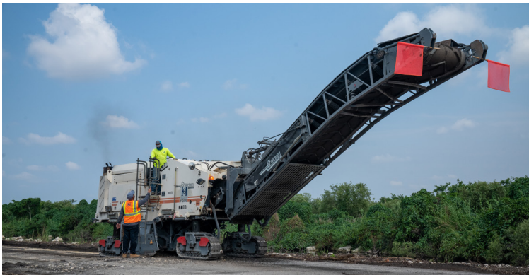
Figure 5. Removing the roadbed of the old Tamiami Trail. (Photo by SFWMD.)
