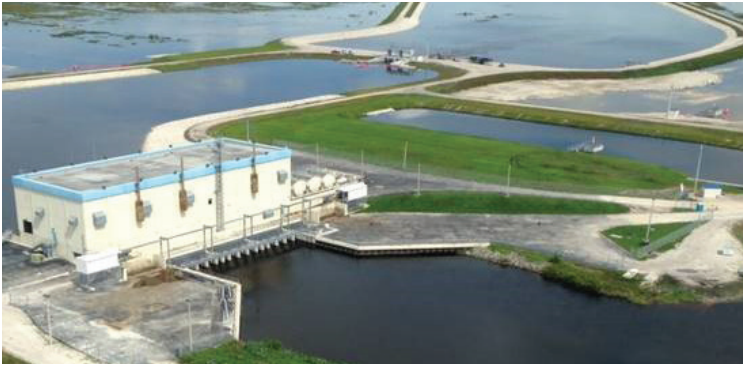
As part of Restoration Strategies, the A-1 Flow Equalization Basin will create 60,000 acre-feet of storage capacity. Construction is complete and operational testing and monitoring have begun.
