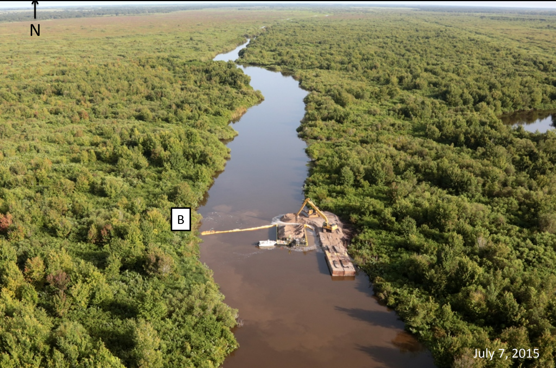
MacArthur Ditch backfilling – initial plug construction
