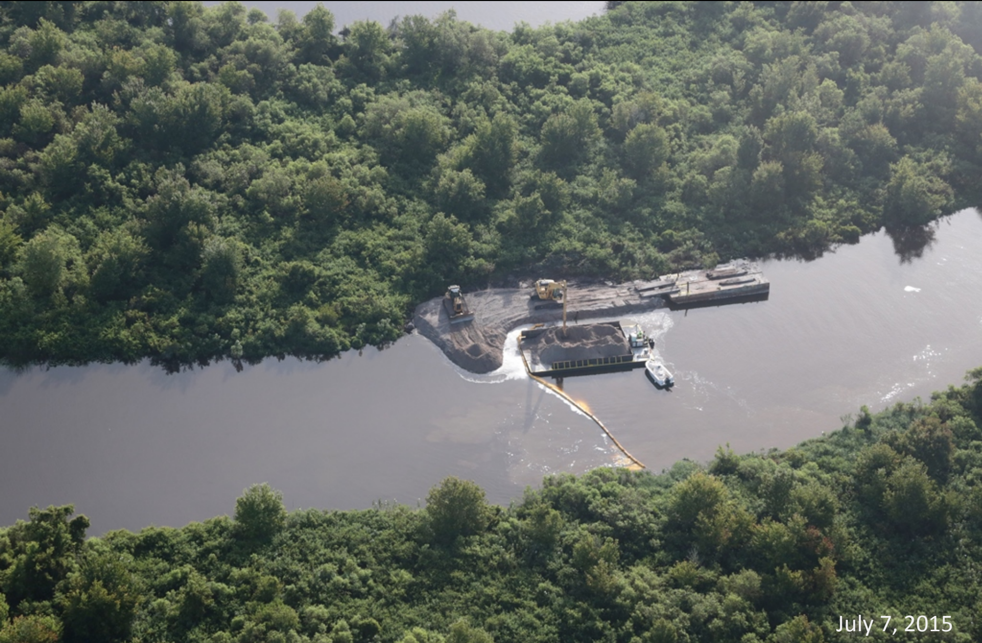
Construction of an initial plug for the MacArthur Ditch backfill. Spoil is being barged in from the south to backfill the ditch.
