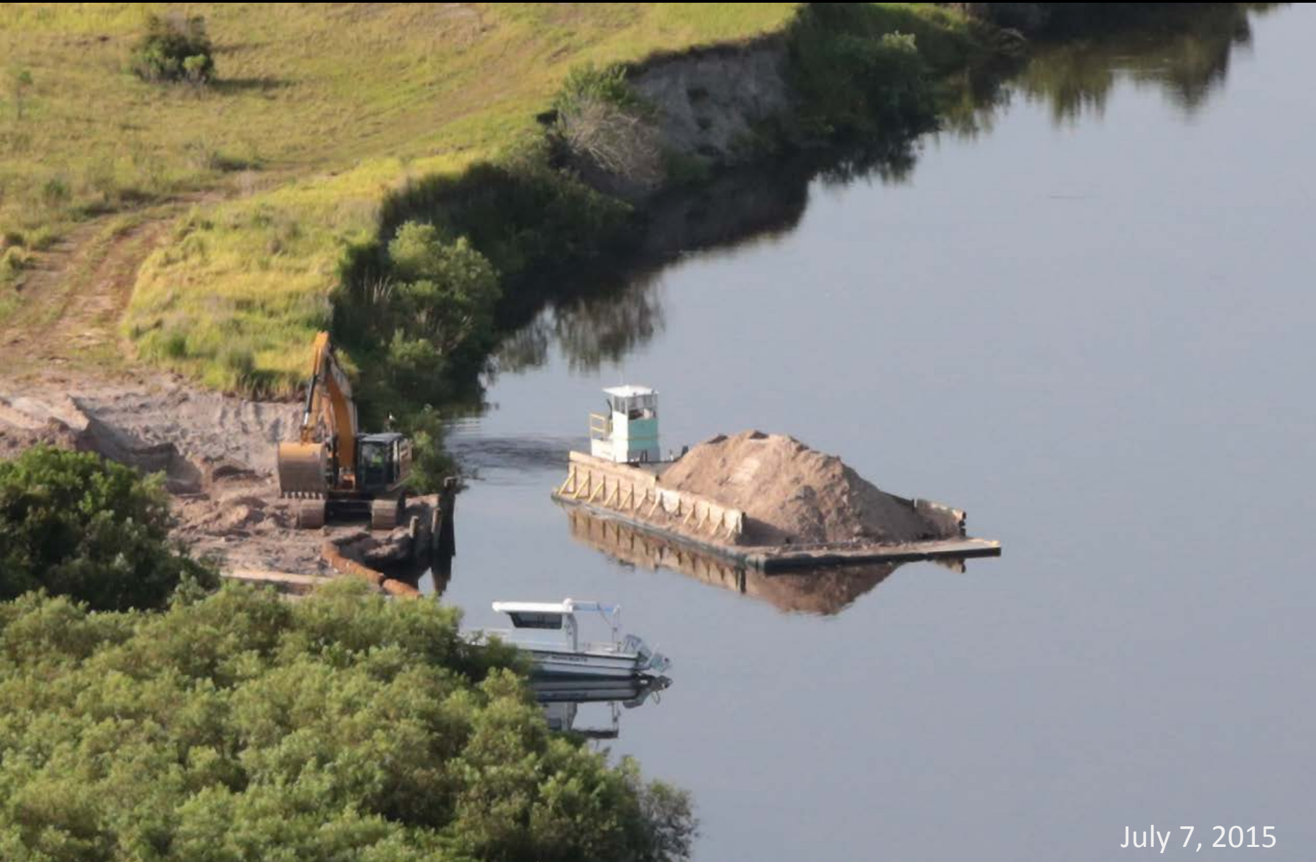
A barge loaded with spoil heads upstream towards the worksite of the MacArthur Ditch backfilling contract, part of the Kissimmee River Restoration Project.
