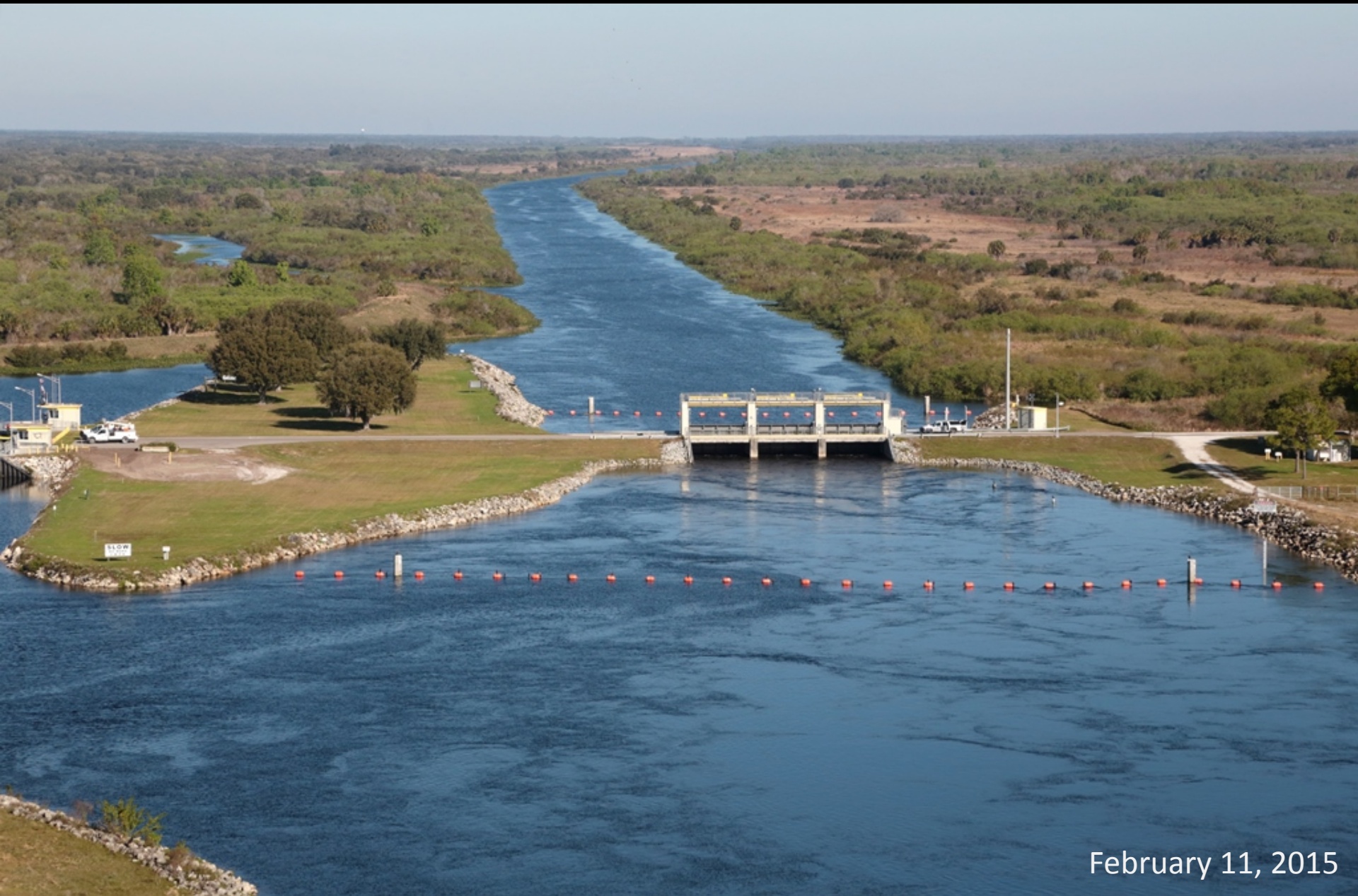
S65A water control structure and C-38 canal (Discharge out of S65A was 5,456 cfs on February 11)
