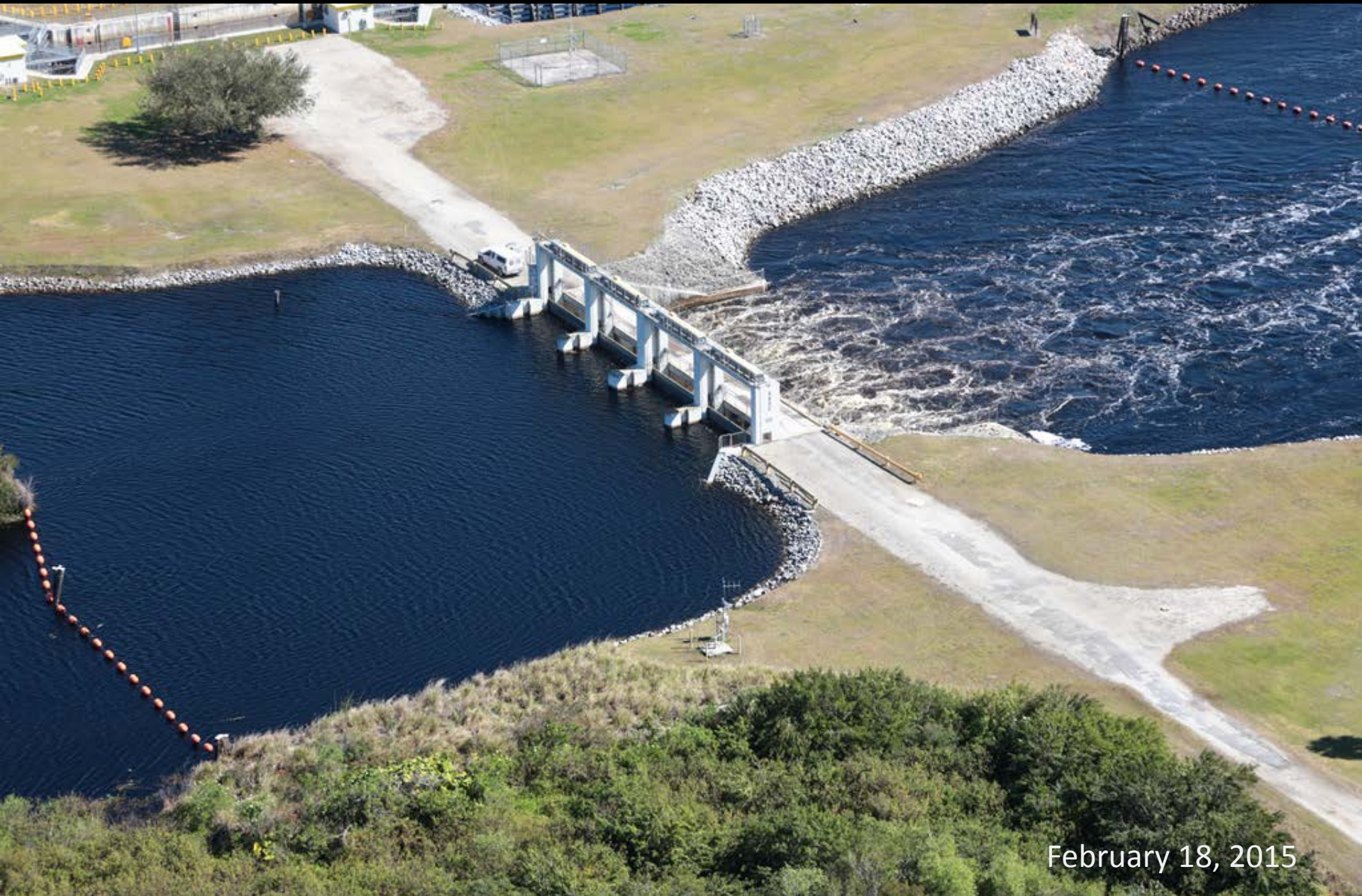
S65C water control structure (Discharge was 5,450 cfs at S65C on February 18)
