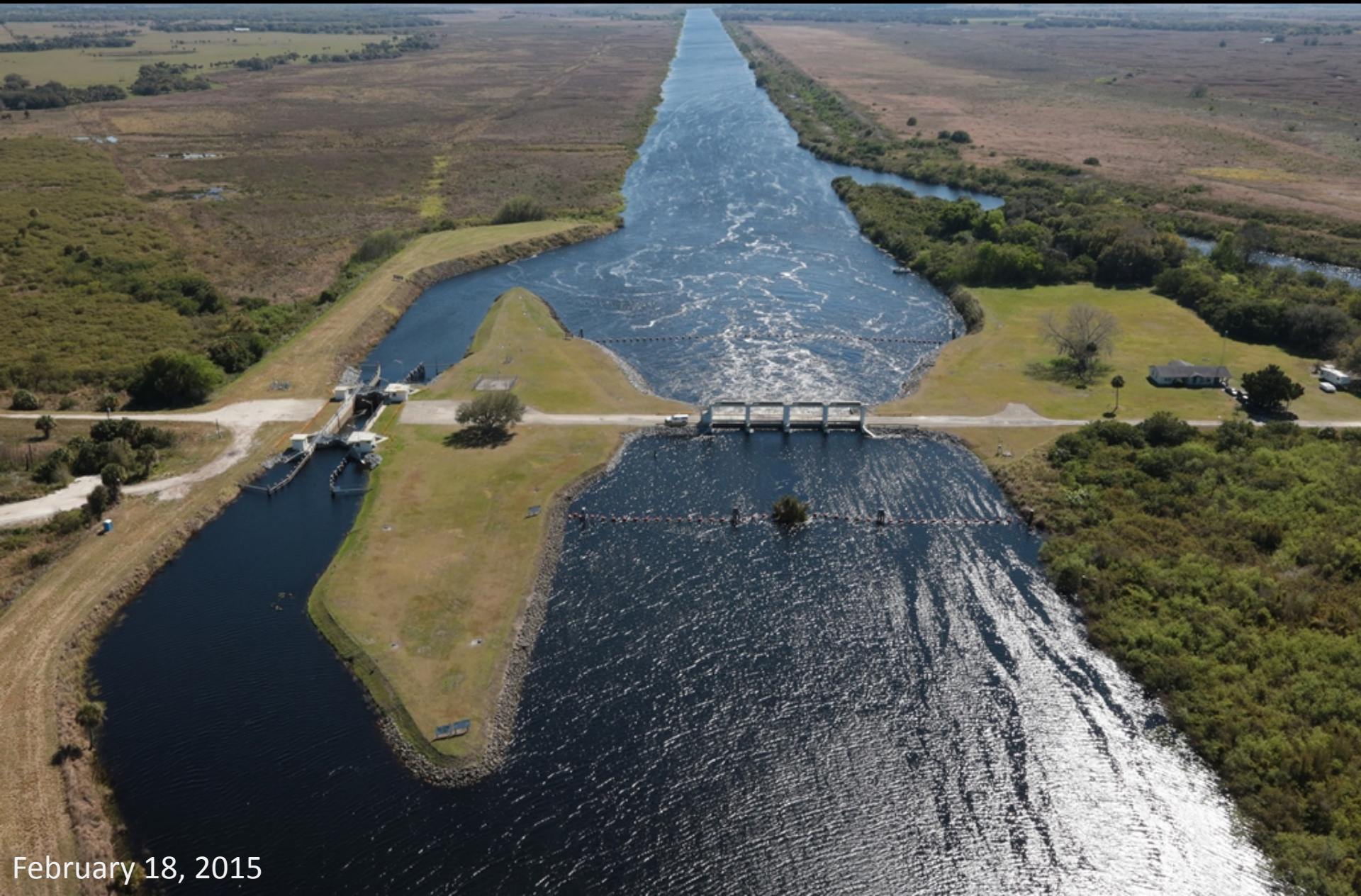
Looking south through the S65C water control structure (Discharge was 5,450 cfs at S65C on February 18)
