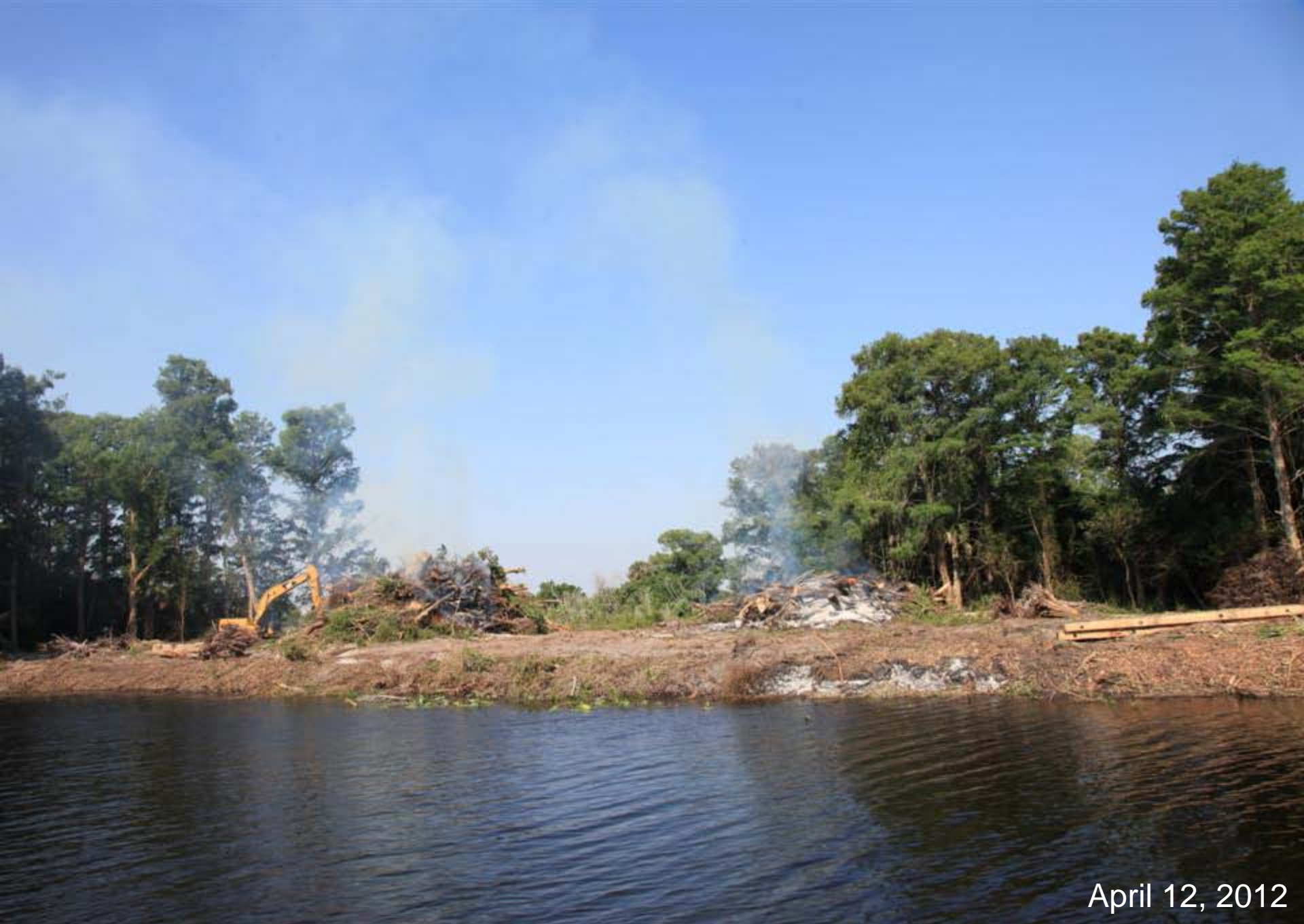
Clearing and grubbing at the 10A reach 3 north site. The last section of river channel recarve for Phase II/III
