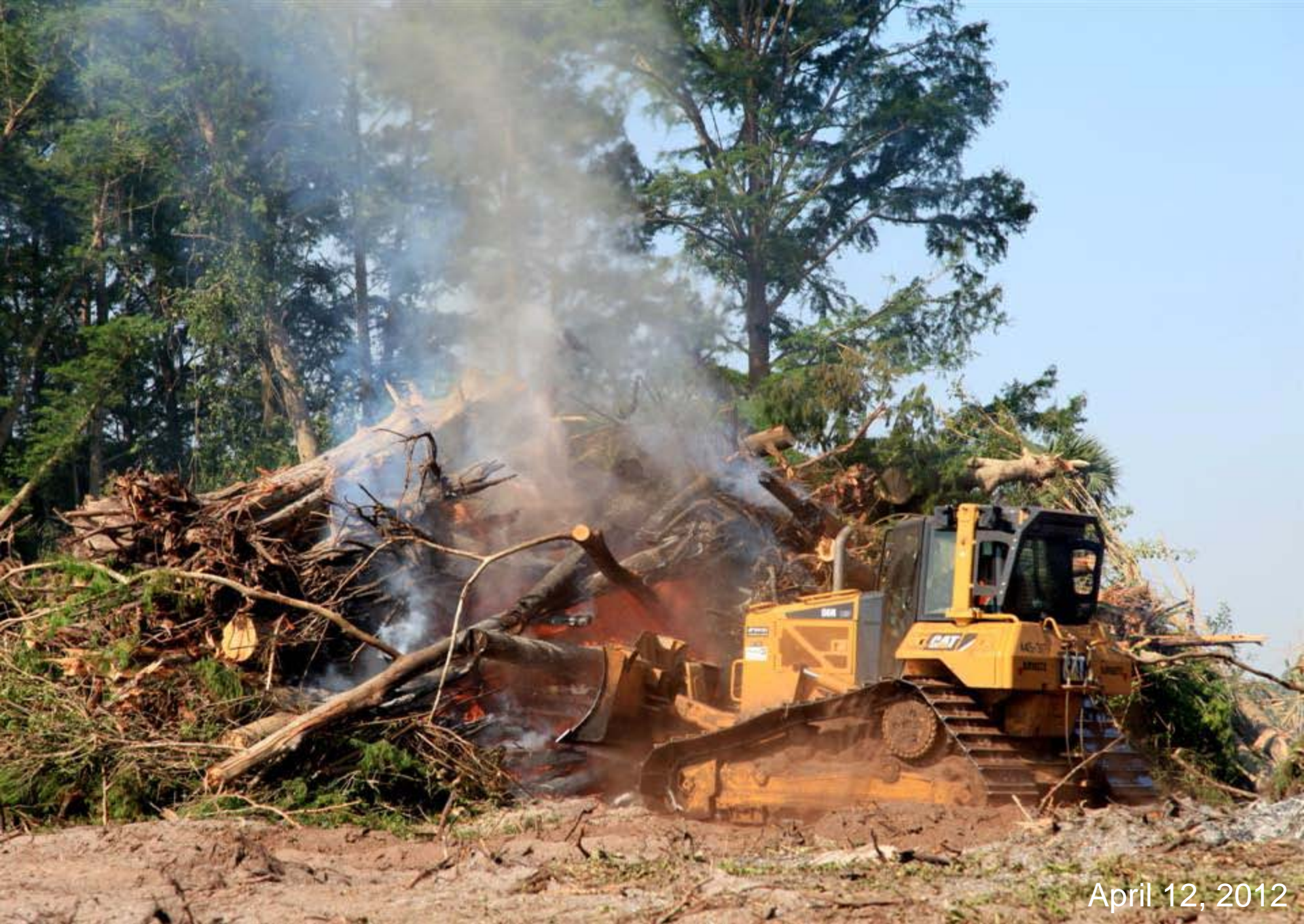
Clearing and grubbing at the 10A reach 3 north site
