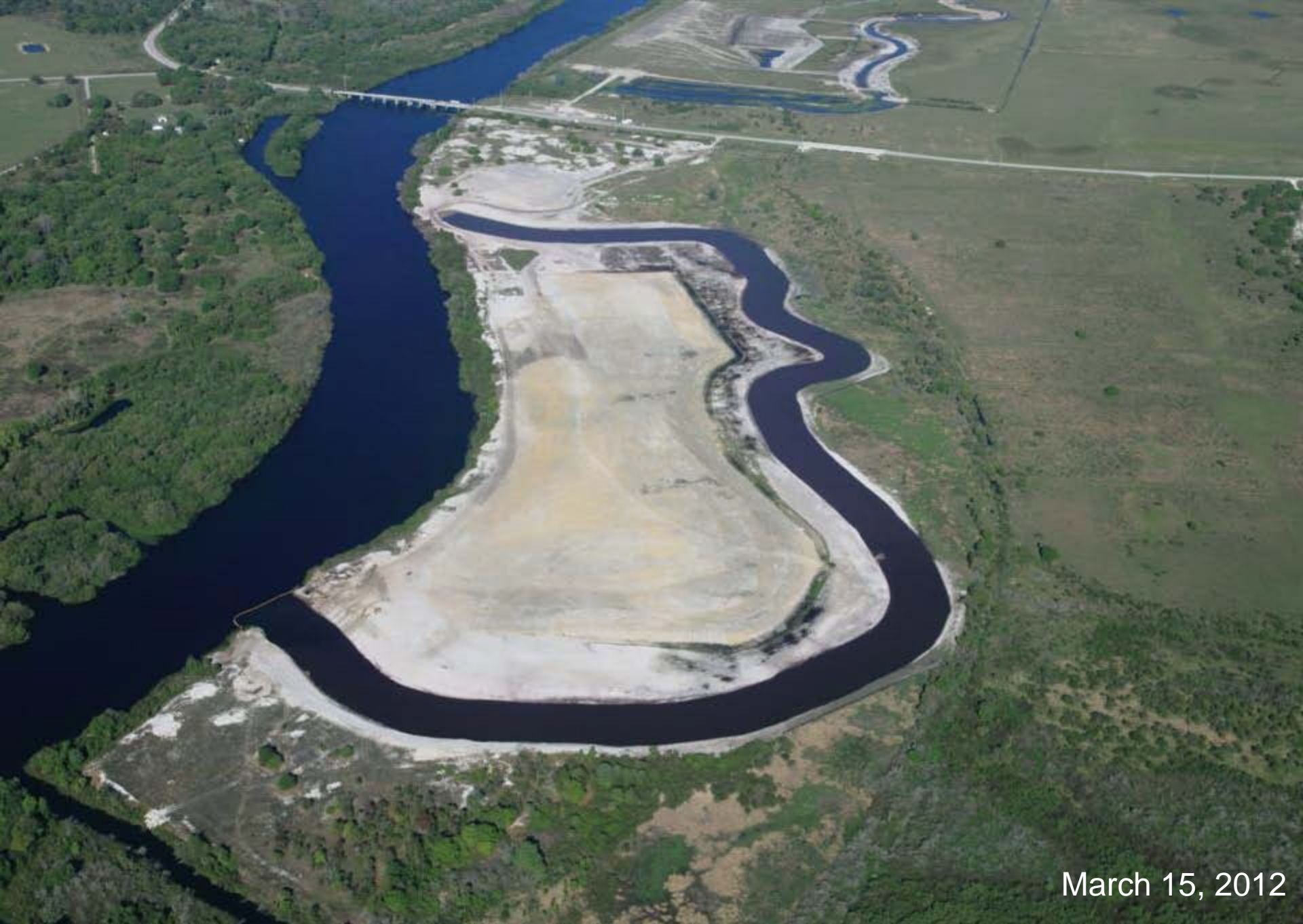
Contract 10A (Reach 3 north) – river channel recarve is complete
