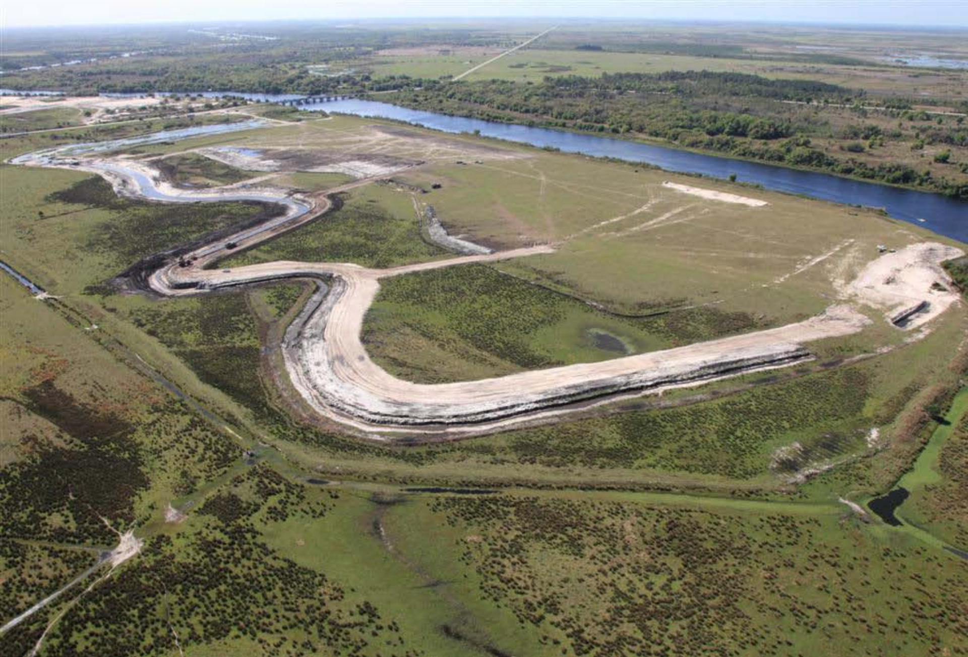
Contract 10A Reach 2 river channel recarve is well underway!
