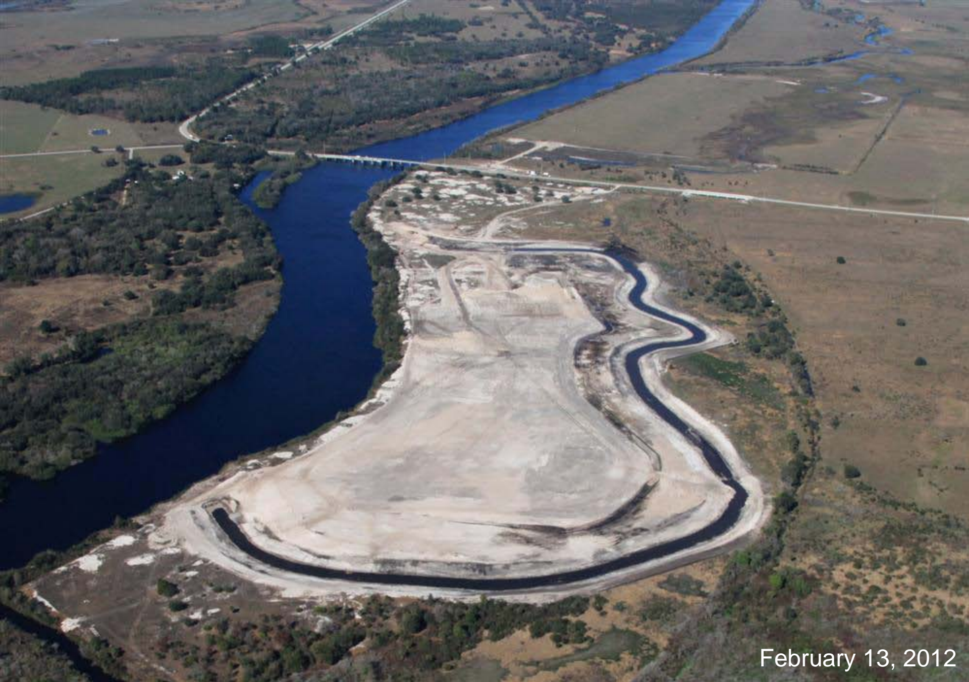
Contract 10A (Reach 3 north) – image from February 2012.
