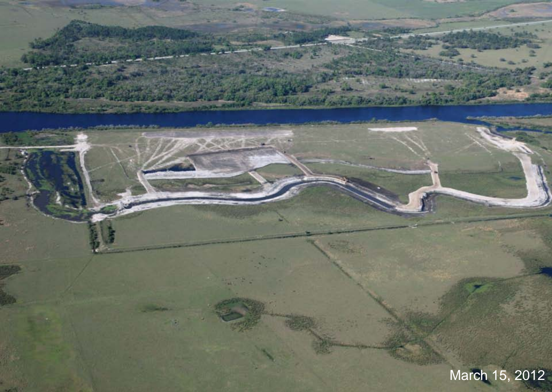
Contract 10A Reach 2 river channel recarve is well underway!
