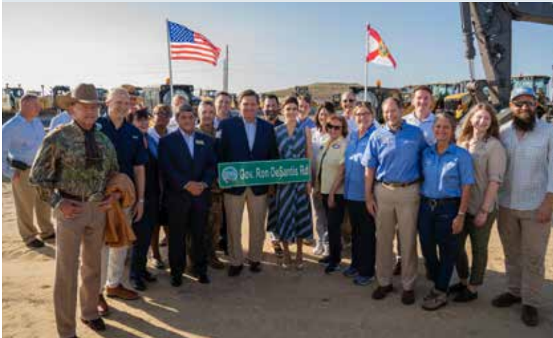
Governor Ron DeSantis, along with state and local officials, breaks ground on embankments and canals to advance the Caloosahatchee (C-43) Reservoir (photo by SFWMD).
