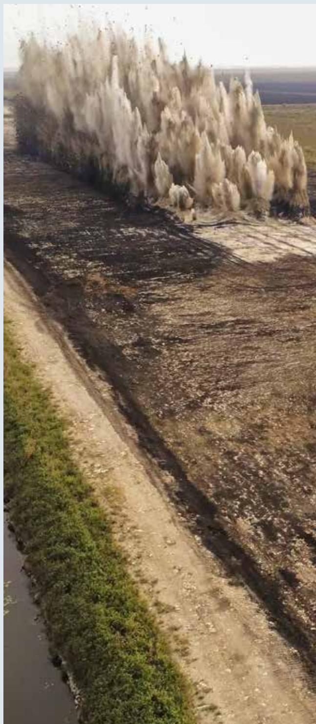
Blasting for the EAA Reservoir Project (photo by SFWMD).
