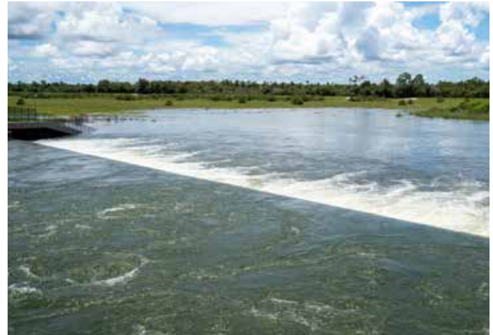
Activation of the Faka Union Pump Station at the Picayune Strand Restoration Project (photo by SFWMD).
