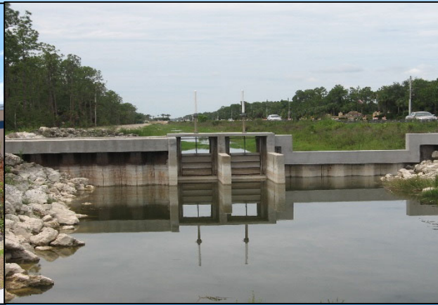
Henderson Creek Structure 2
