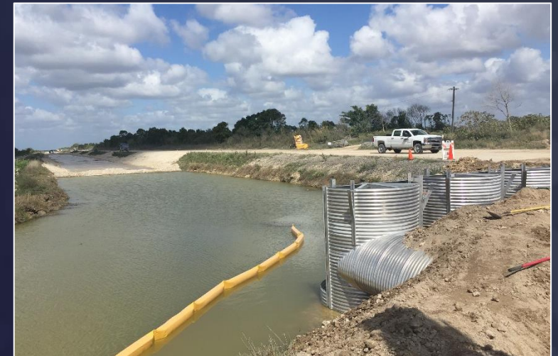
Culverts from C-200 to L-31W Canal
