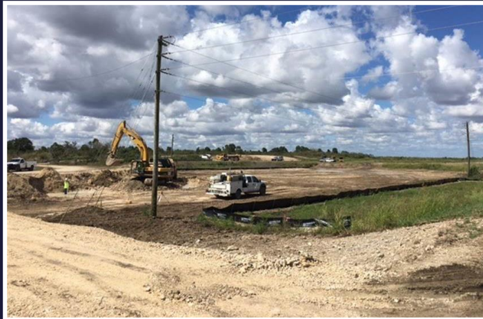
Scraping to Cap Rock and Excavating Sump Area
