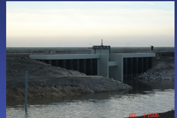
G-396A Control Structure
