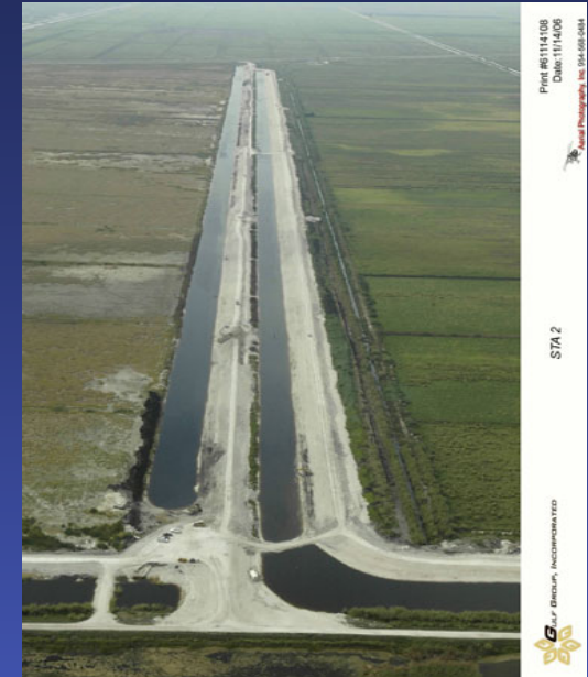
North Levee & Inflow Canal
