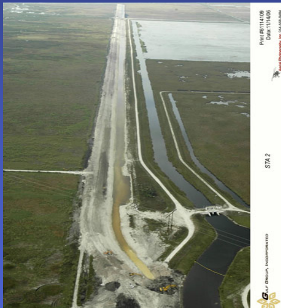
South Levee & Discharge Canal
