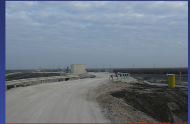
G-342E Inflow Control Structure
