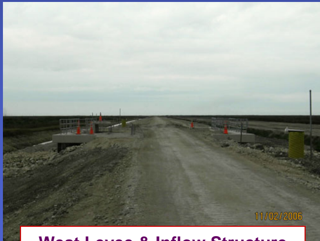
West Levee & Inflow Structure
