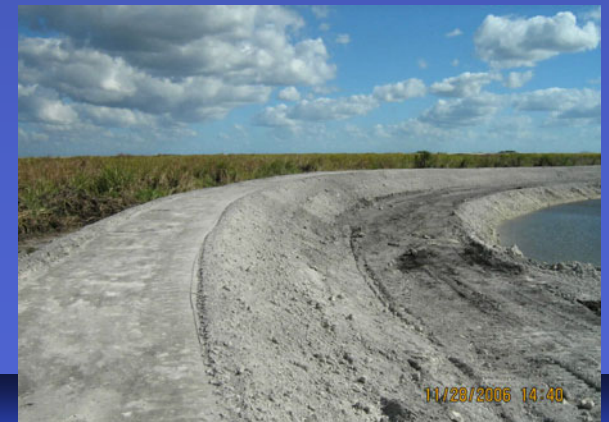
Berm Final Lift
