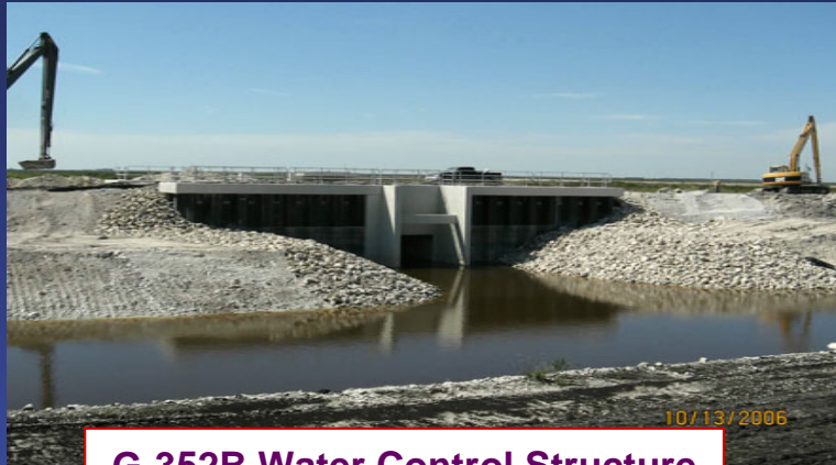
G-352B Water Control Structure
