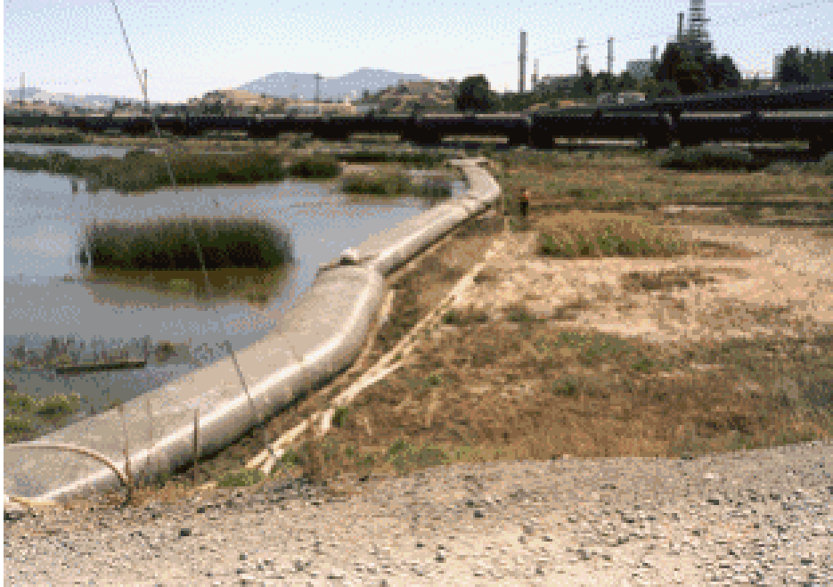
Figure 4. Aquadam® installation along a wetland boundary
