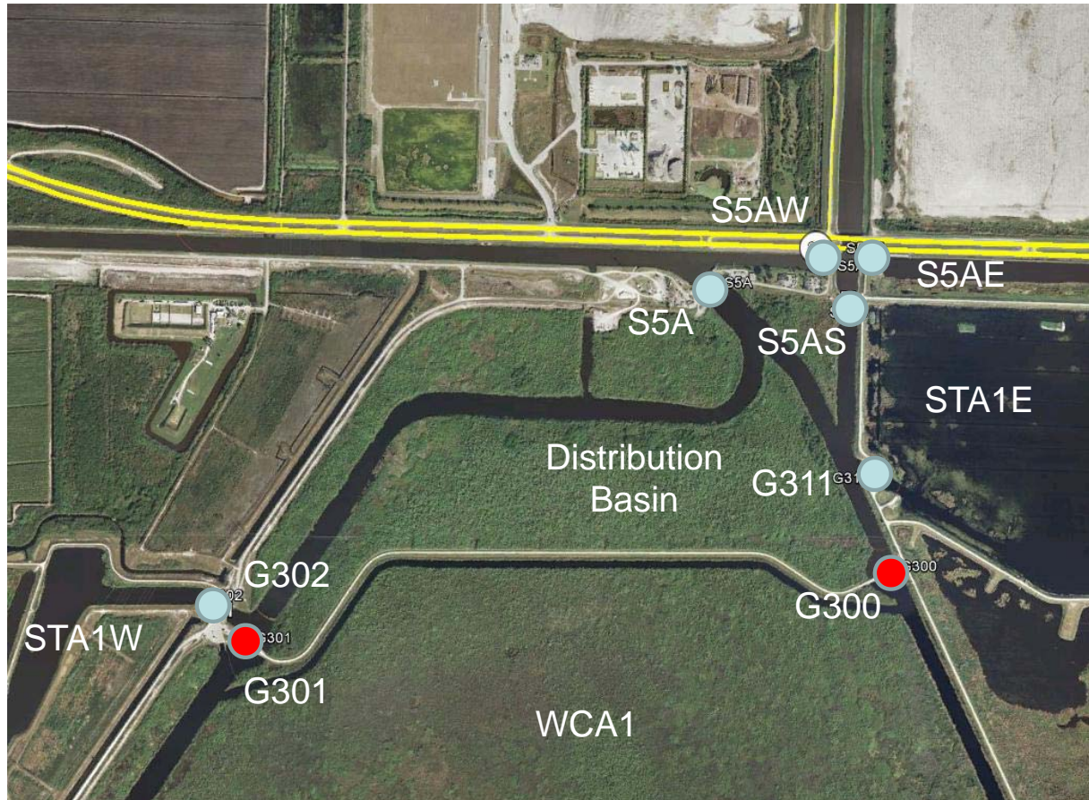
S5A and Associated Structures Showing G300 and G301
