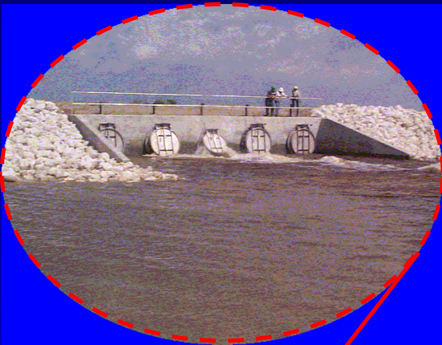
S-332B Looking North-East
