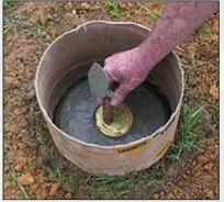
Bronze or Brass disks set in poured-in-place concrete, or existing structure with a deep foundation.
