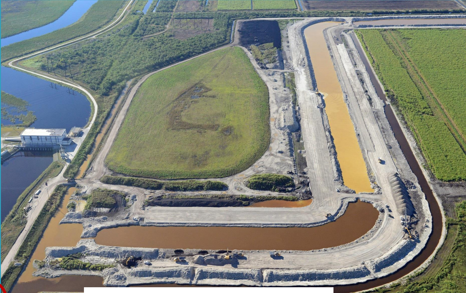
Canal and Embankment Construction
