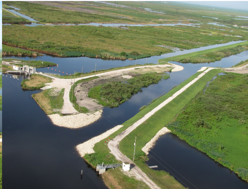
New Western Flow-Way Inflow Canal & Cell 5A Embankment
