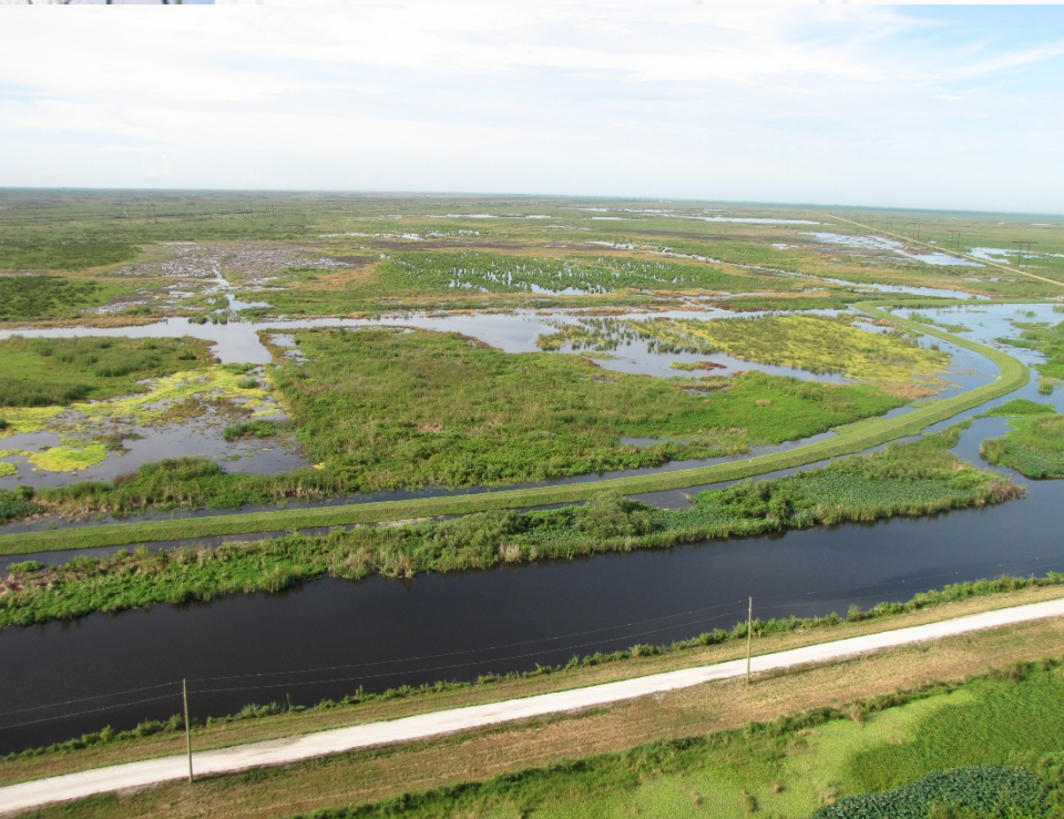
New Western Flow-Way Inflow Canal & New Cell 1A Embankment
