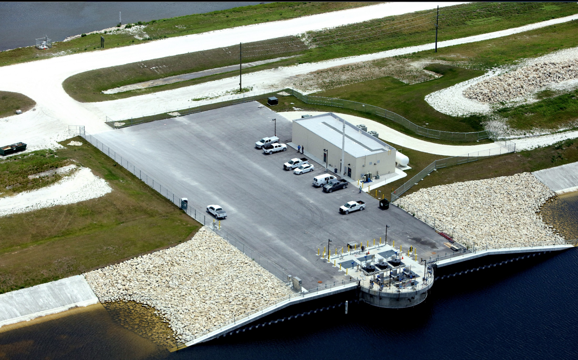
G-539 Pump Station
