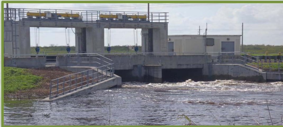
STA-1W G-303 gated structure
