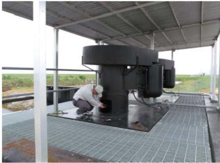
Figure 3. Making tachometer reading on Pump #2 impeller shaft.
