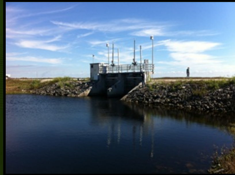
Typical Stem Operated Slide Gate
