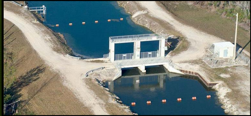
Typical 2 Bay Gated Spillway
