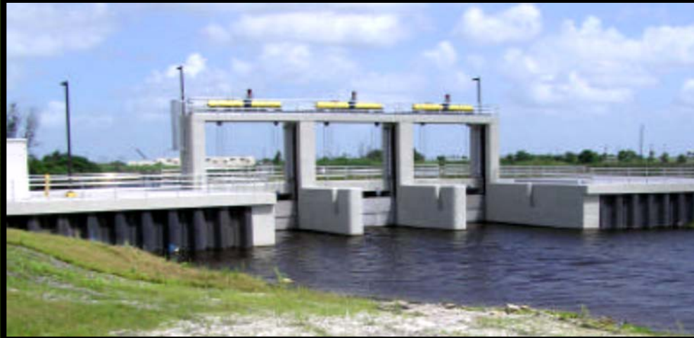
Typical 3 Bay Gated Spillway
