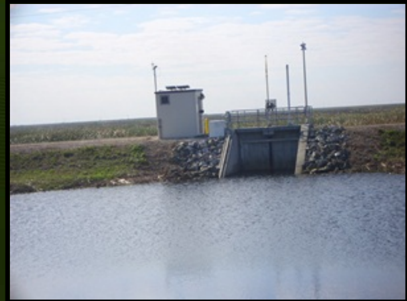
Typical Stem Operated Slide Gate
