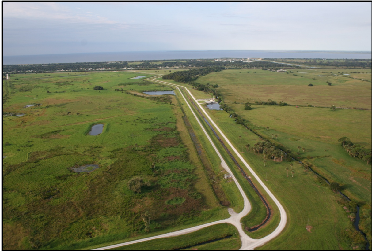
Oblique photo showing the stormwater treatment cell (east side, top; west side, bottom)
