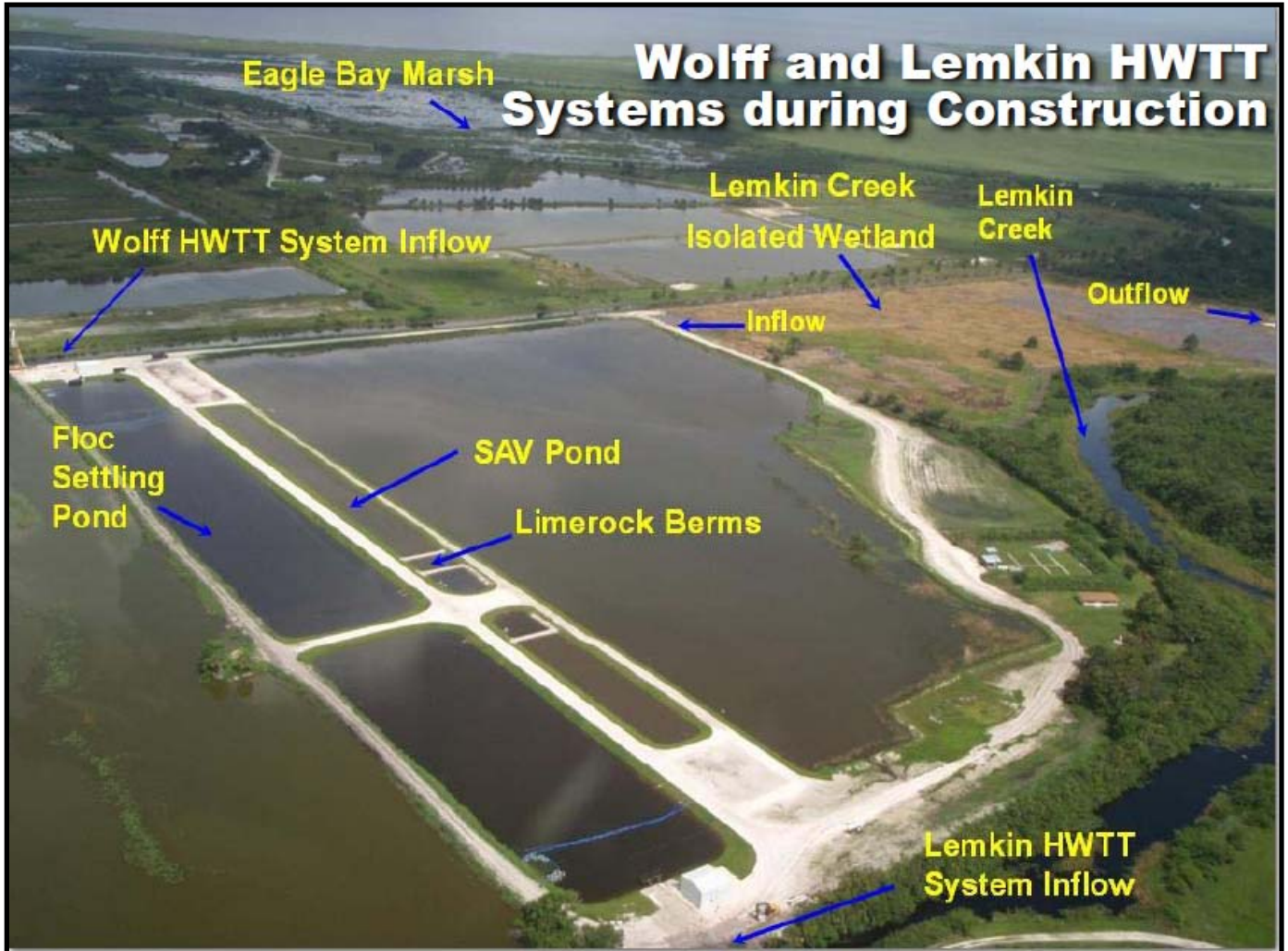
An oblique Aerial showing the Lemkin Creek water treatment facility, and its components
