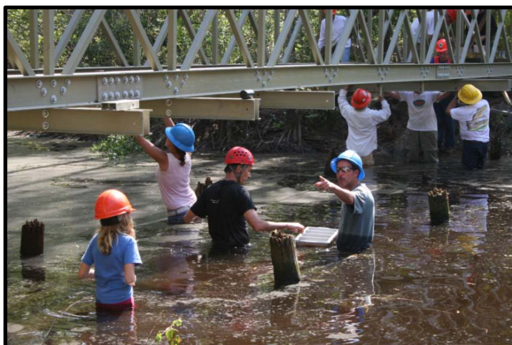
The Florida National Scenic Trail runs through KICCO, and is maintained by Florida Trail Association volunteers. Here a group of volunteers assembles and installs a bridge over Tick Island Slough. The materials for the bridge was purchased by the District.
