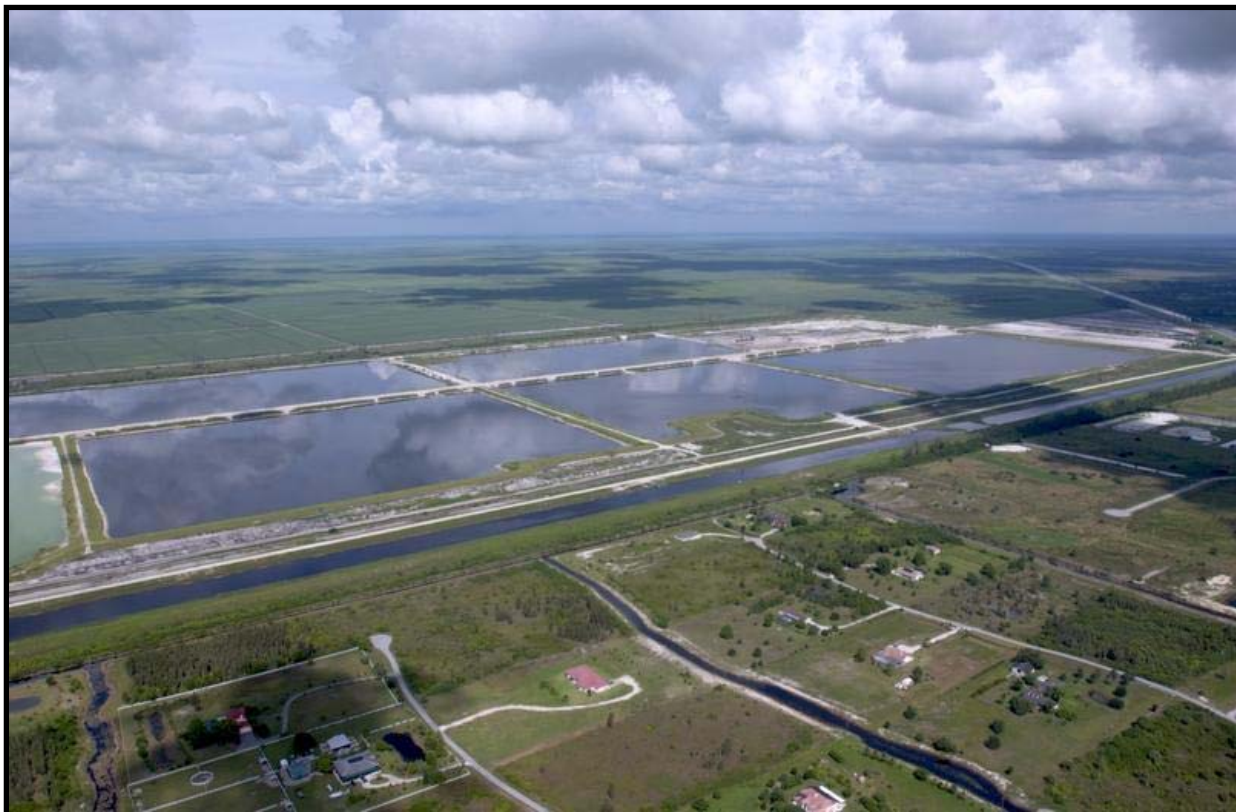
Oblique photo showing the L-8 Reservoir.
