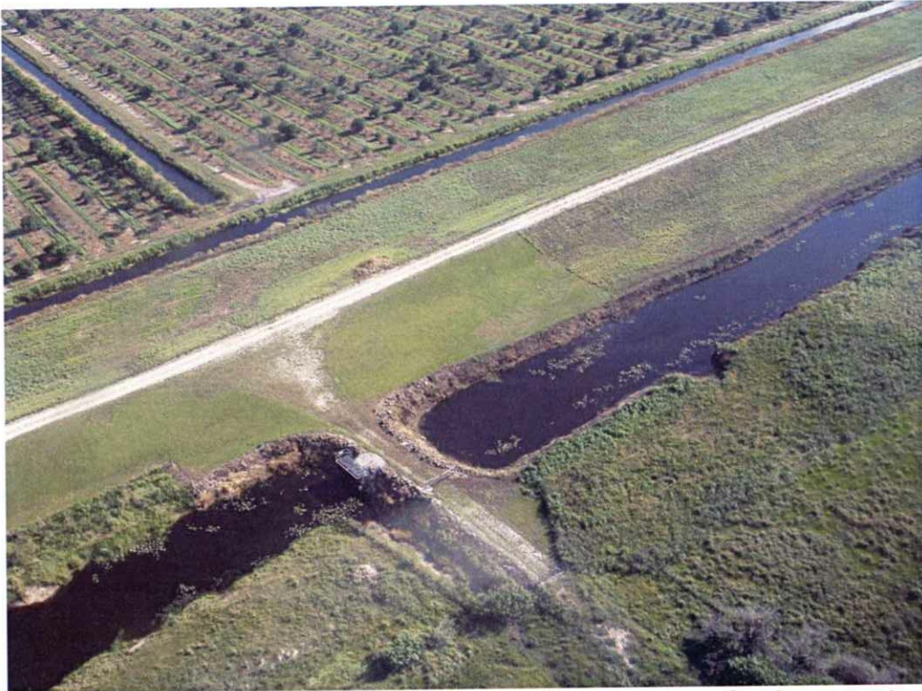
G-96 structure at the northwest corner of the Jackman Cattle property
