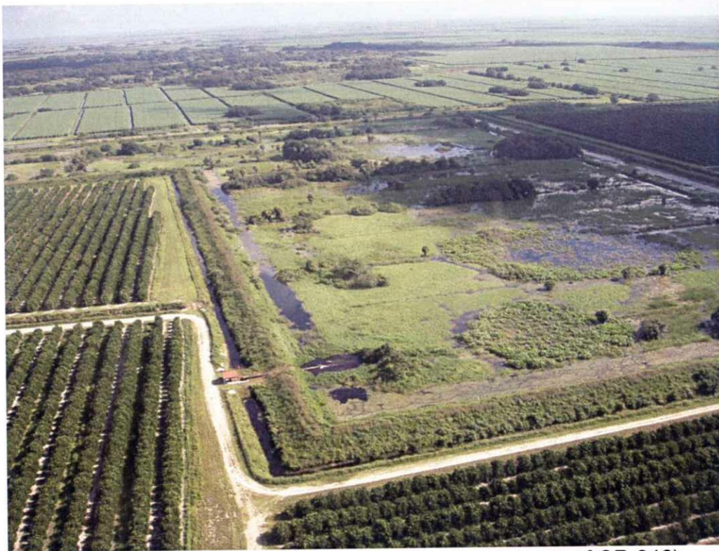
Reservoir for Basin 26-323-05 (ALICO property east of CR 846) Looking North
