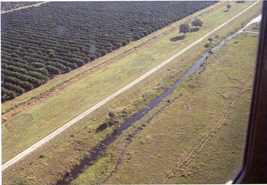
Constriction in the L-1 Canal along the north boundary of the 26-303-01 basin
