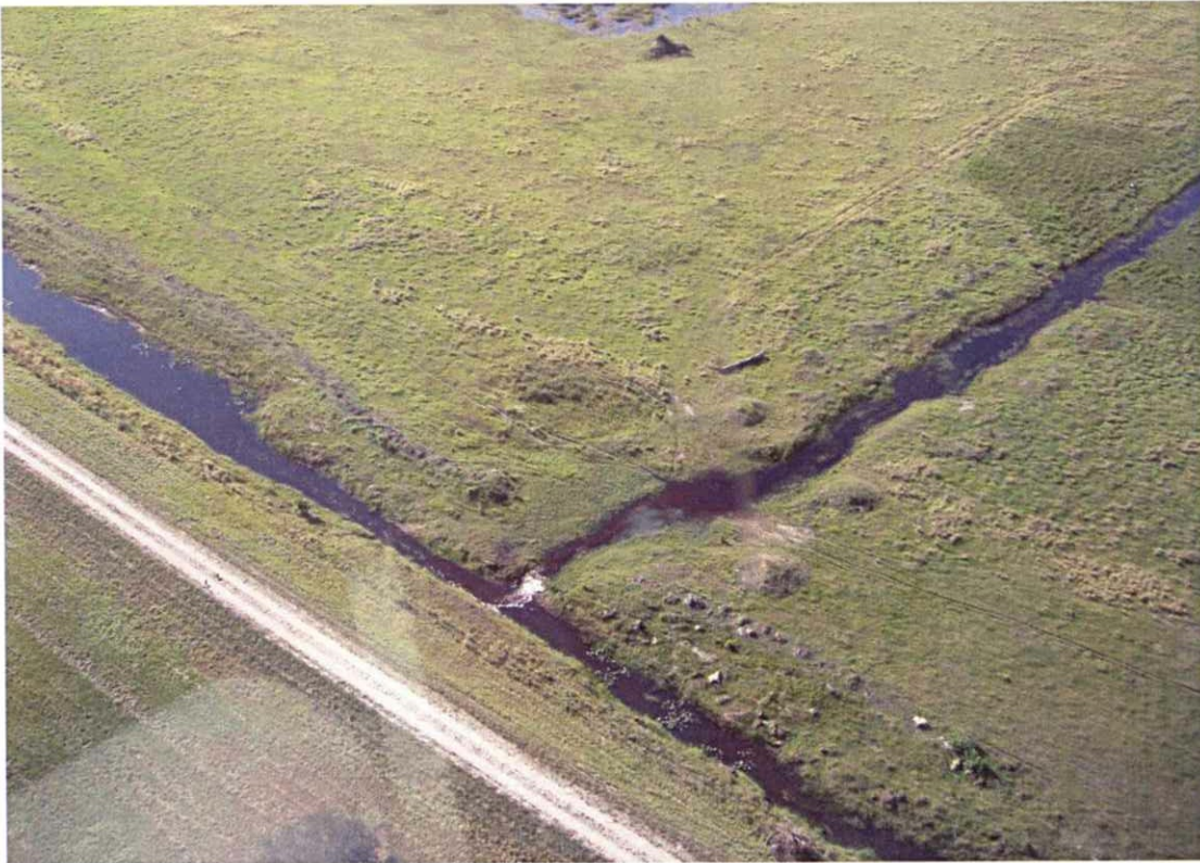
Field ditch drainage for the 26-303-01 basin
