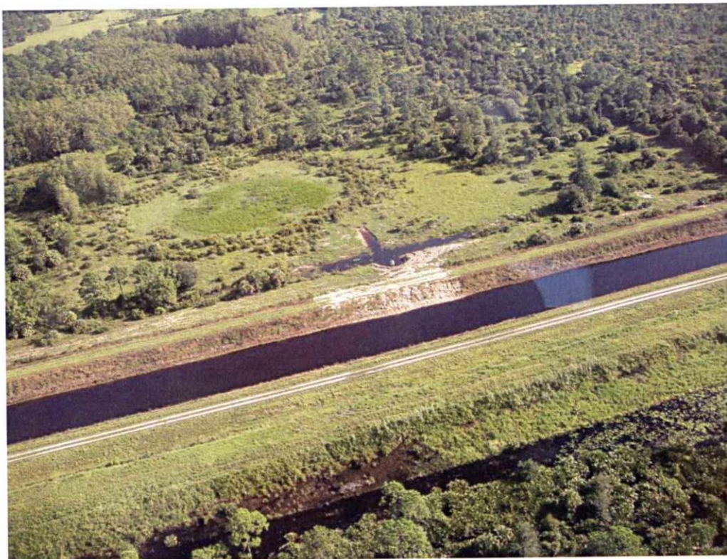
L-2W Canal Looking North – Outflow structure from Basin 26-322-3 (top) and reservoir for Basin 26-323-1 (bottom)
