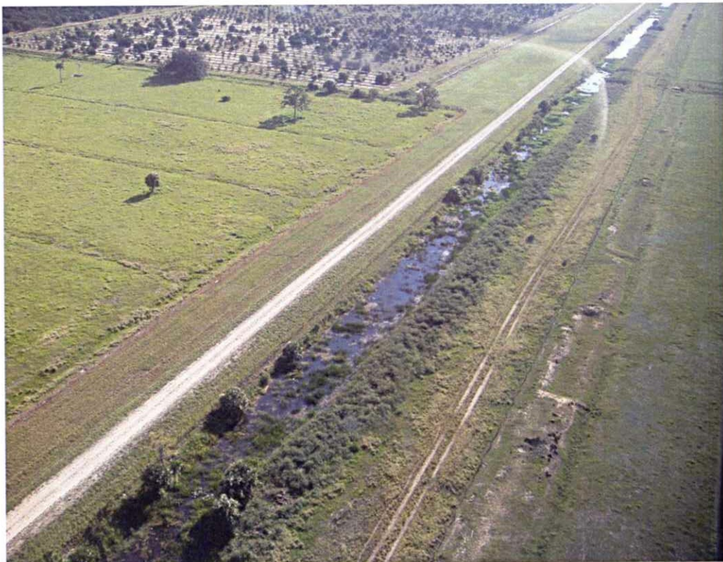
Vegetation growth in the L-1 Canal along the north boundary of the 26-303-01 basin
