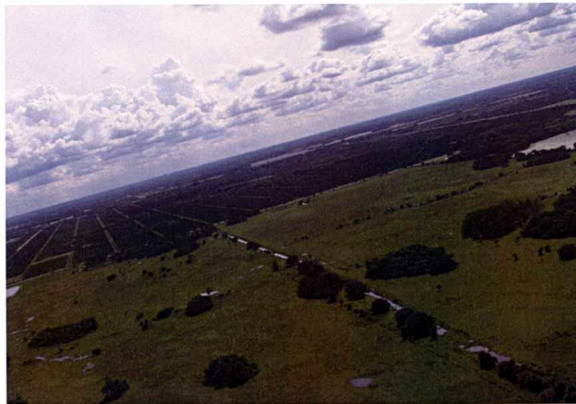
Looking southwest from Basin 26-314-01 at Basin 26-306-01 along the main drainage canal that crosses CR 833 and follows north and western perimeter of the property discharging into the Deer Fence Canal
