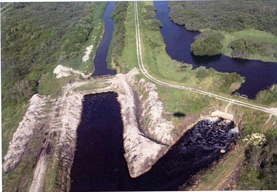
G-152 Structure – Looking west ALICO Basin 26-323-01 (left) and Central County Drainage District reservoir (right) (NOTE: Ditch between structures was installed by SFWMD to act as a barrier to ALICO Basin 26-323-01)
