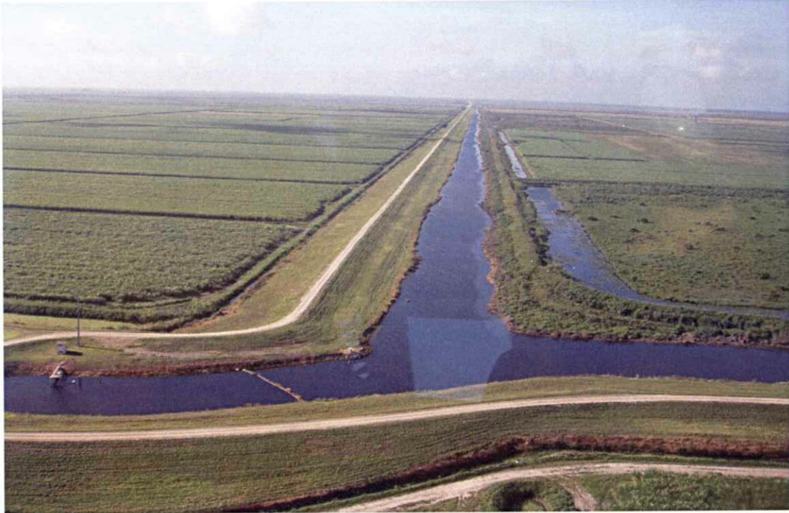
L-1 Borrow Canal – Looking south with the northeast Jackman Cane and Cattle reservoir on the right
