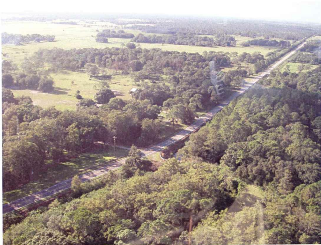
G-135 at the Northwest corner of the 26-303-01 basin – Looking Southeast
