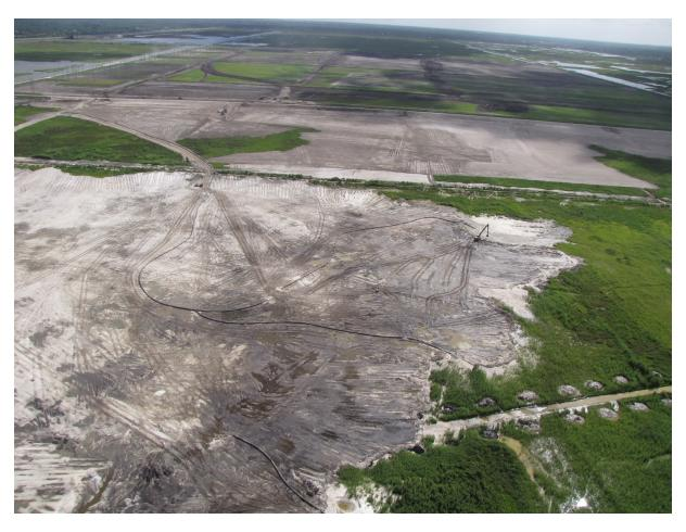
Earthwork for STA-1E Improvements. Photo illustrates the re-distribution of fill dredged from WDC in Cell 7. The regrade of Cell 5 can be seen in the background
