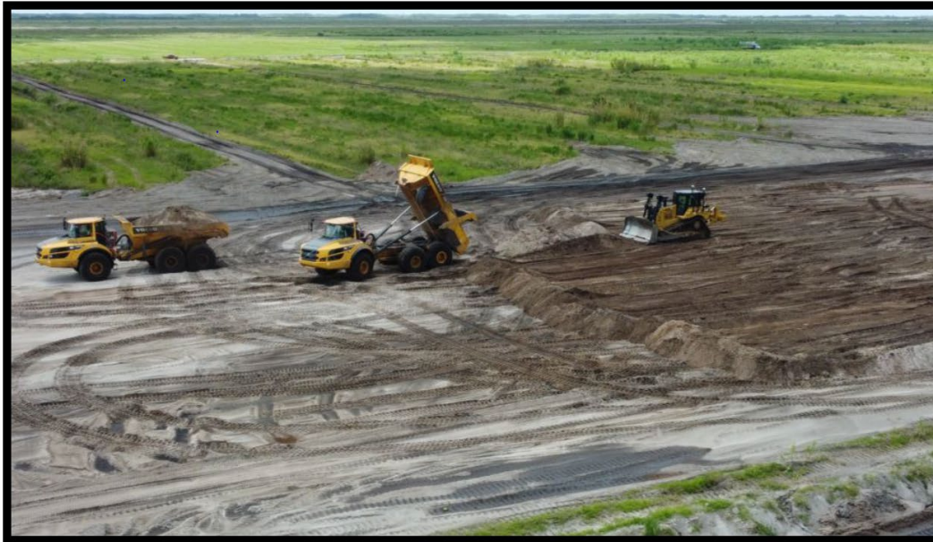
C-139 FEB perimeter levee construction.
