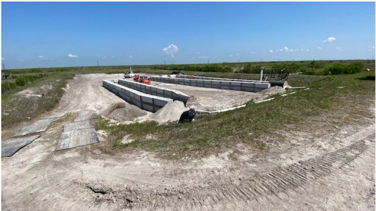
Landscape study. STA-1W south Test Cell 13. Installation of two 80-foot flumes .
