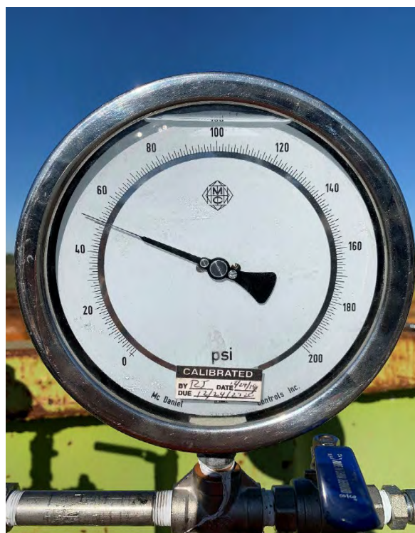
Figure 10. Calibrated Pressure Gauge at beginning of casing pressure test.
