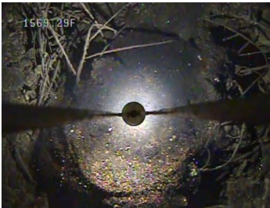
Figure 5. Blockage at 1,570 ft bpl with partial cavern floor.
