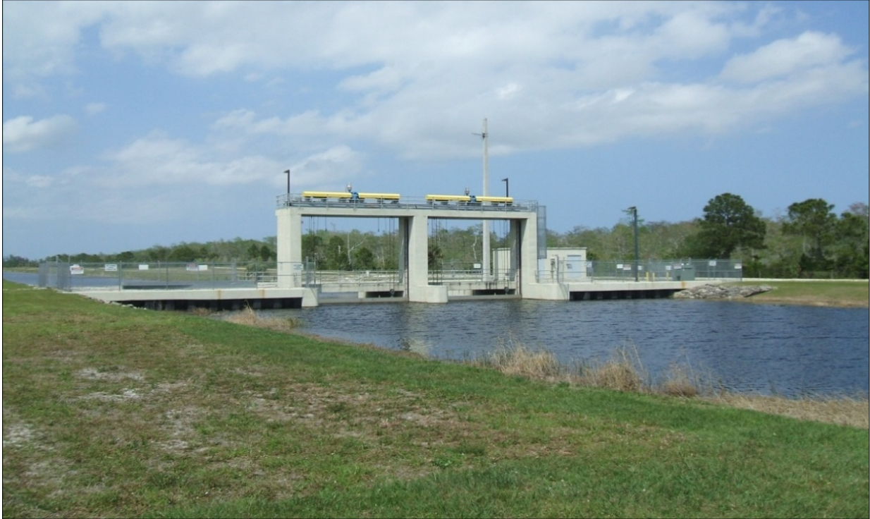
Figure 2. G-160 water control structure in the C-18 Canal.
