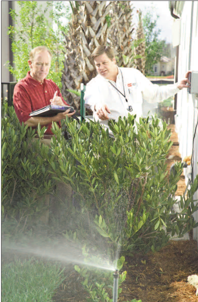
Simple steps, such as checking the alignment of sprinkler heads, can improve the efficiency of automatic irrigation systems and ensure the right amount of water goes where it is needed.
