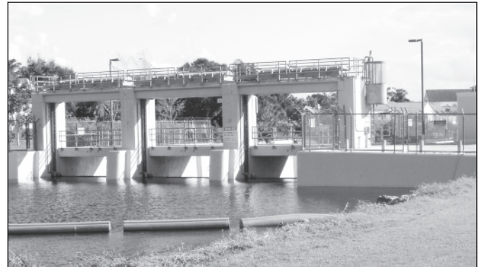
Bank erosion on the Hillsboro Canal contributes to the buildup of sediment around coastal structures, such as the G-56 (above) located on the eastern end of the canal just west of Military Trail.
