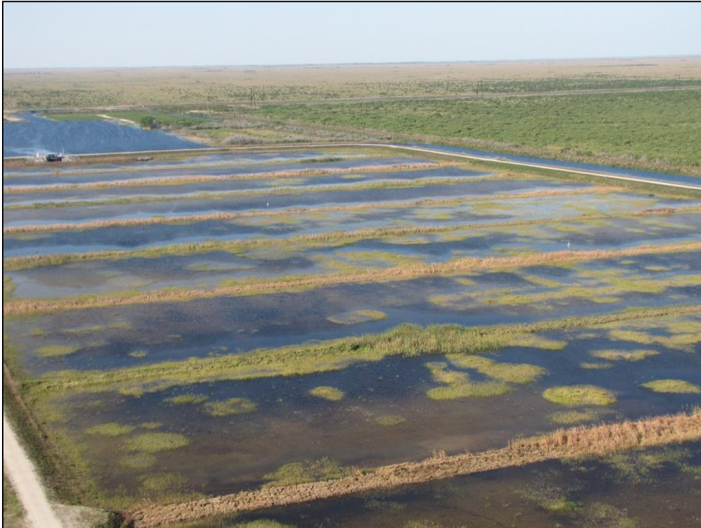
Figure 4-4. Aerial photo of the outflow region of the PSTA Cell in STA-3/4, showing several emergent vegetation strips and the outflow pump structure G-388. The vegetation on six of the twelve strips in the PSTA Cell was treated with herbicide in April 2012, then compacted to minimize hydraulic resistance during hydraulic (pulse) events conducted in July–August and October 2012.
