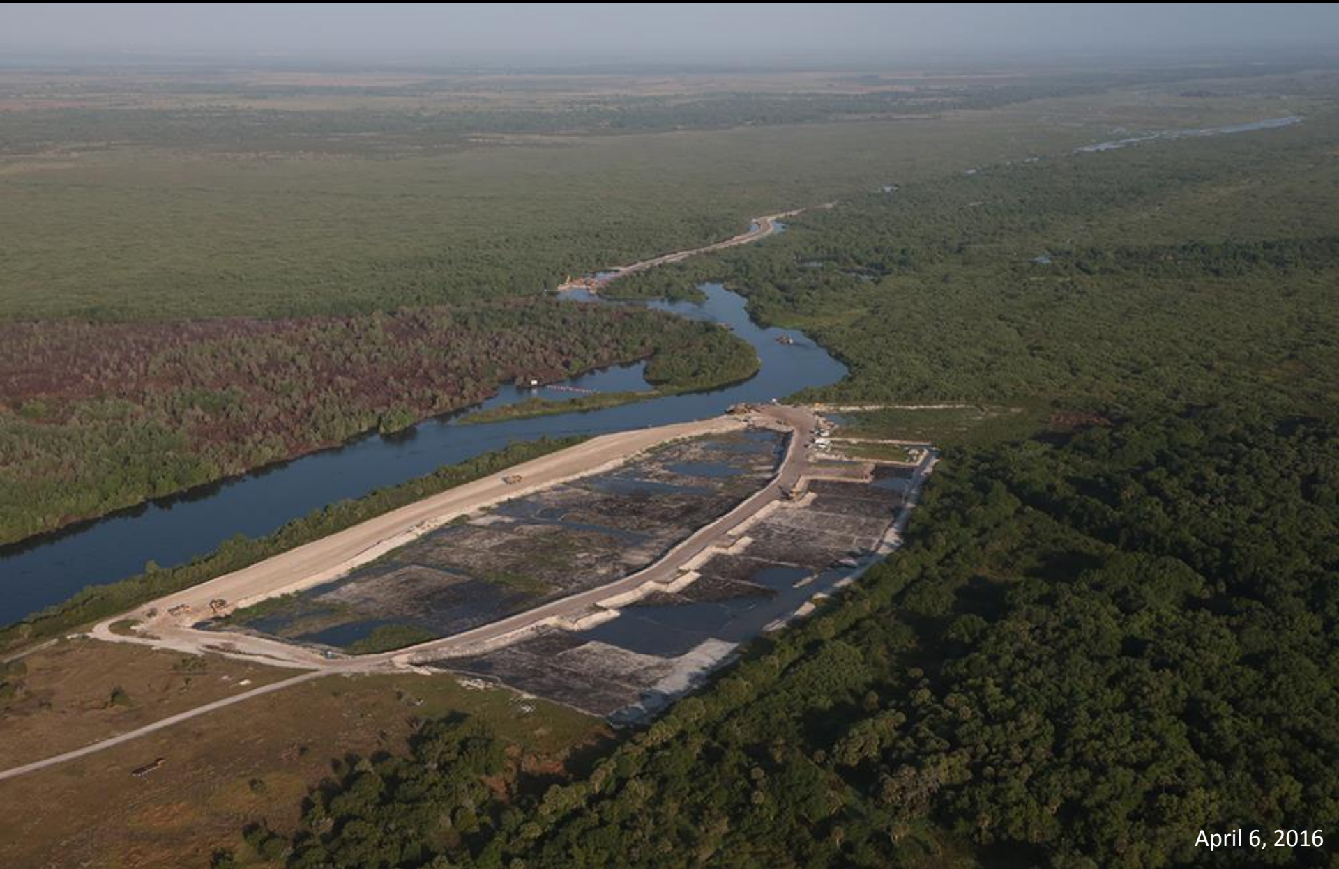
Looking northwest at the MacArthur Ditch backfill and borrow area. Spoil is excavated from the borrow area and barged upstream to backfill the ditch to the north.
