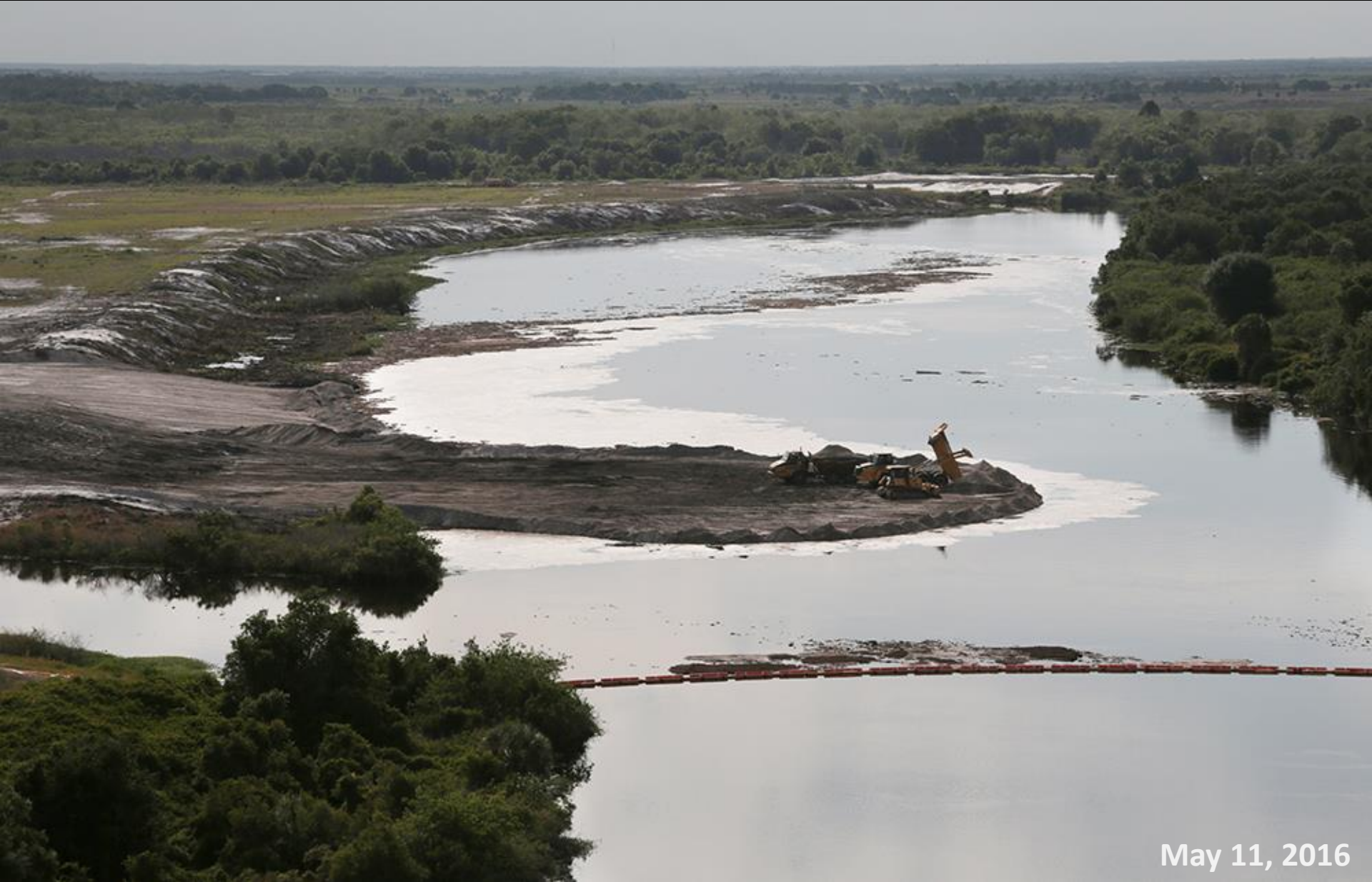
Kissimmee River Reach 3 restoration area looking south down the C-38 canal where a plug is being placed at the north end of reach 3 just south of the HW98 bridge.
