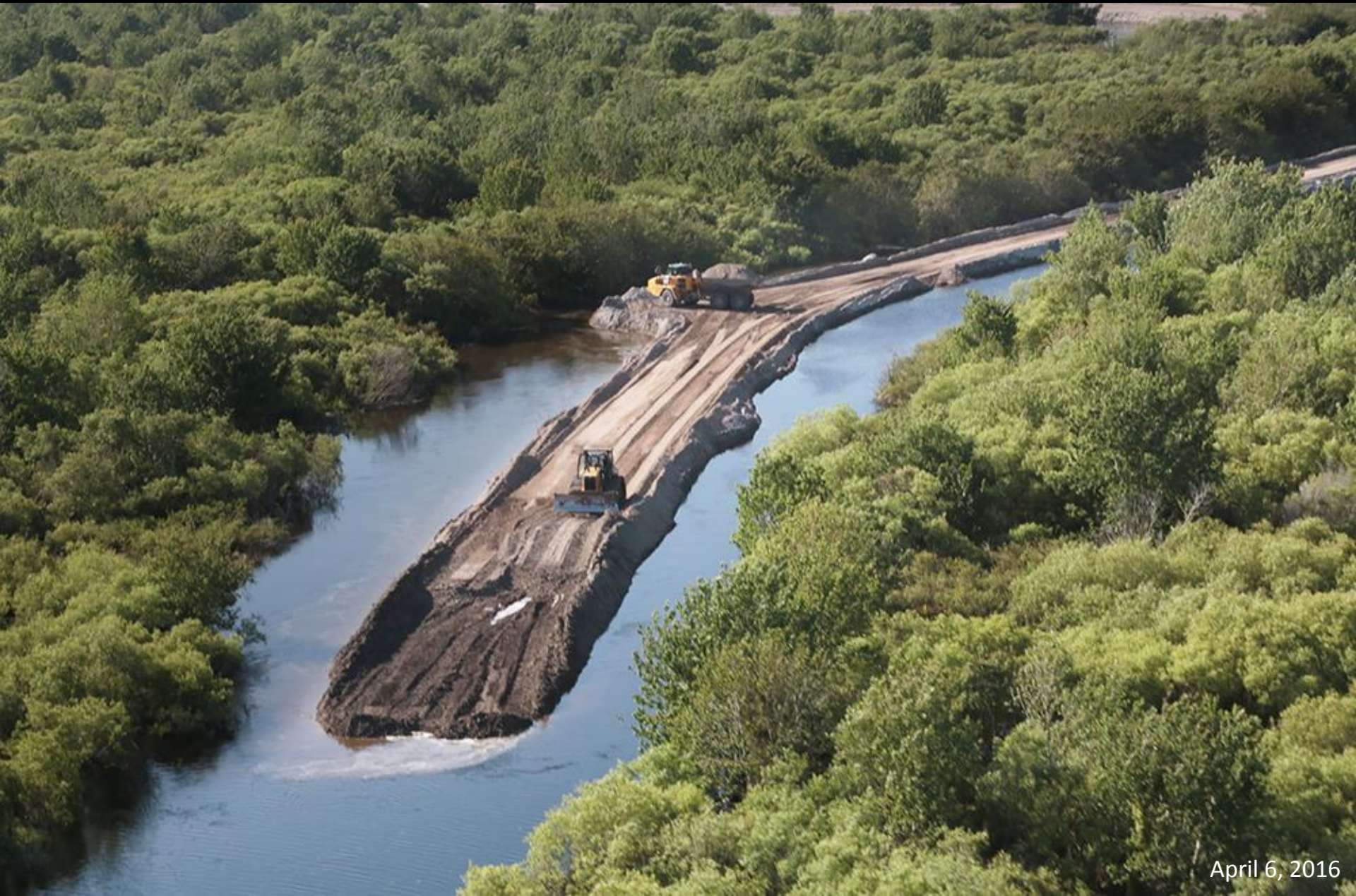
Backfilling the MacArthur Ditch.
