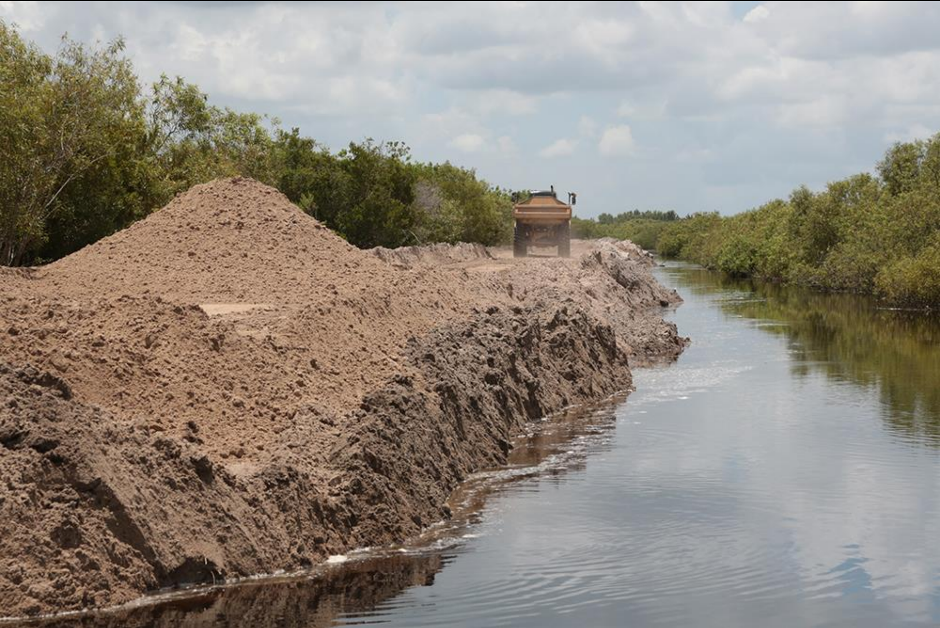
Backfilling the MacArthur Ditch.
