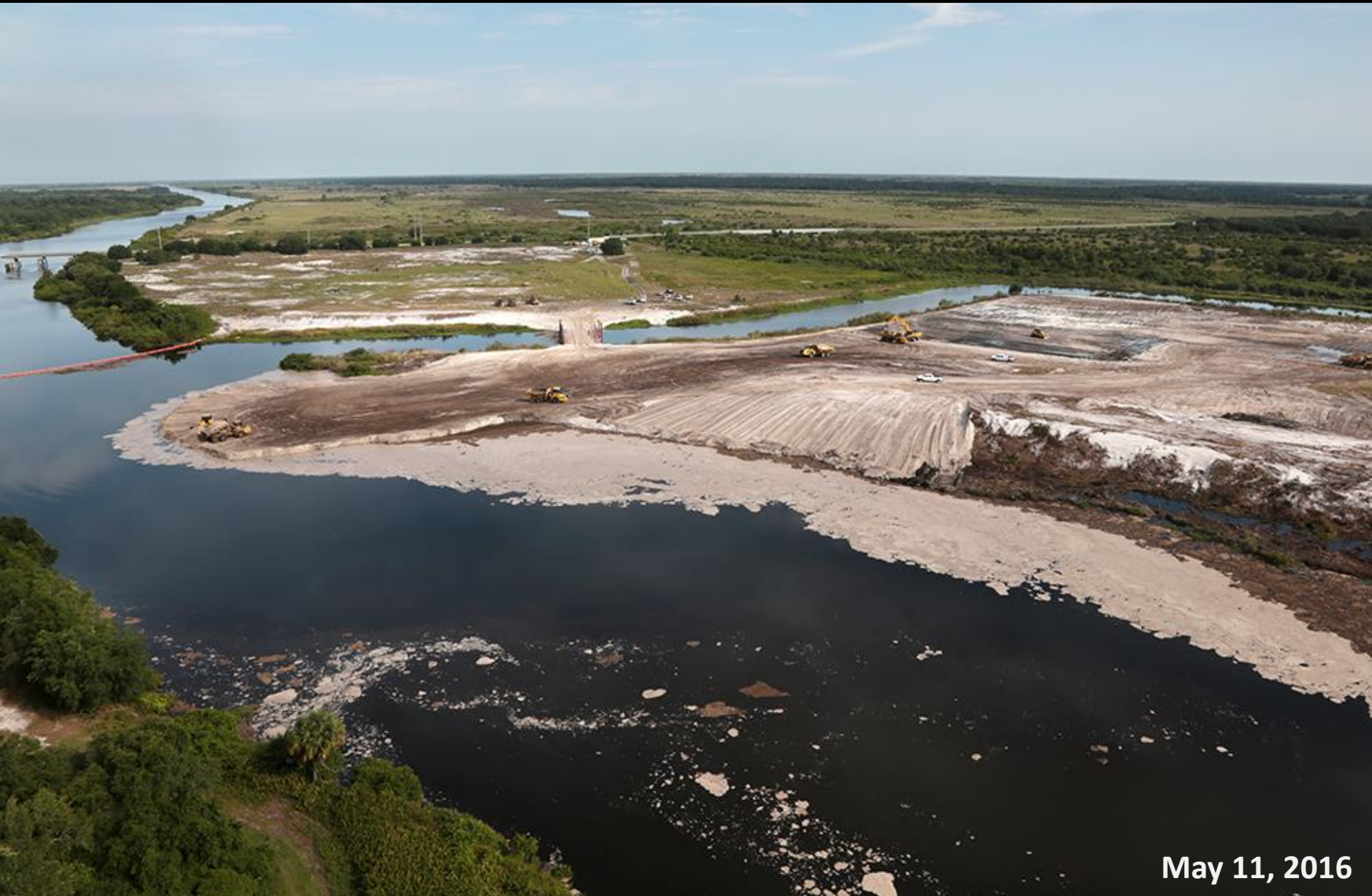
Kissimmee River Reach 3 restoration area looking north up the C-38 canal where a plug is being placed at the north end of reach 3 just south of the HW98 bridge.
