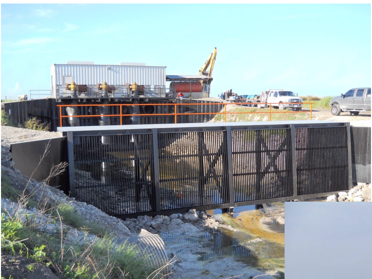
Above: Trash rack to catch canal debris Right: Removal of sediments and vegetation from canals
