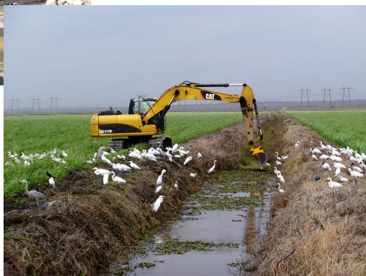
Above: Trash rack to catch canal debris Right: Removal of sediments and vegetation from canals
